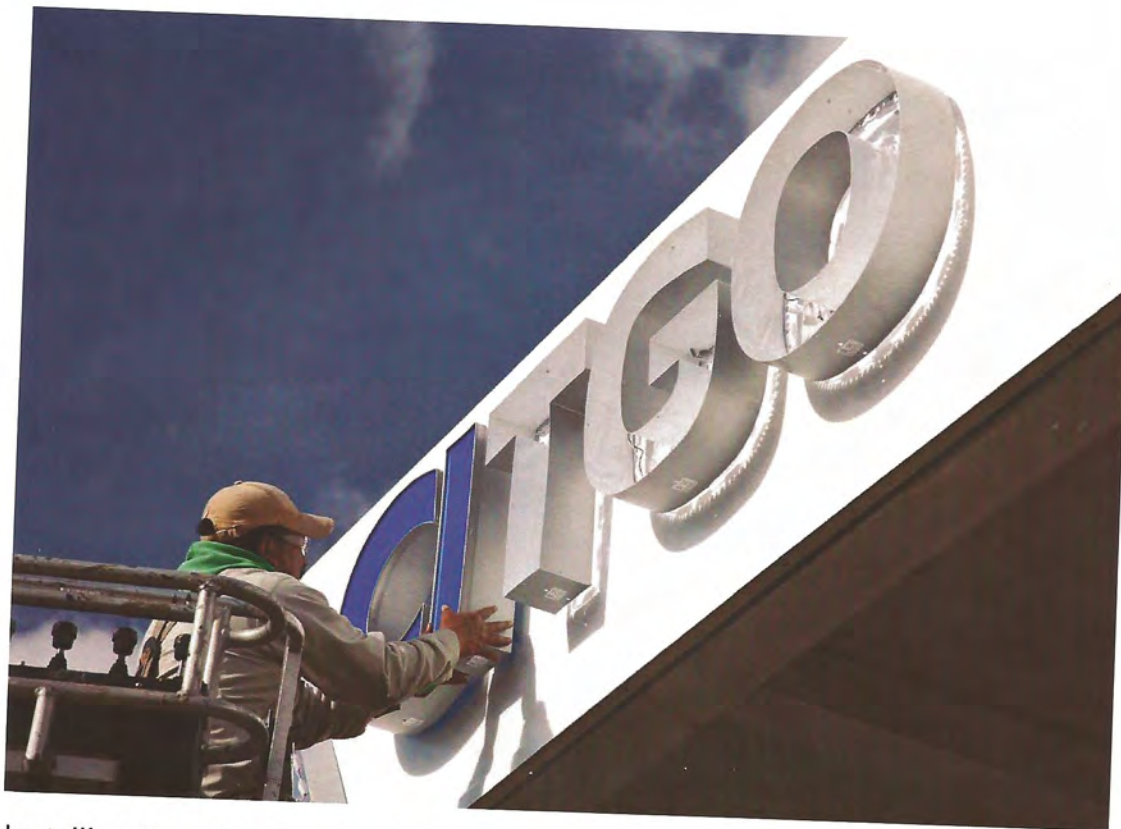
Installing the primary CITGO channel letters. Note the spacers that provide the rear halo effect on these channel letters.
