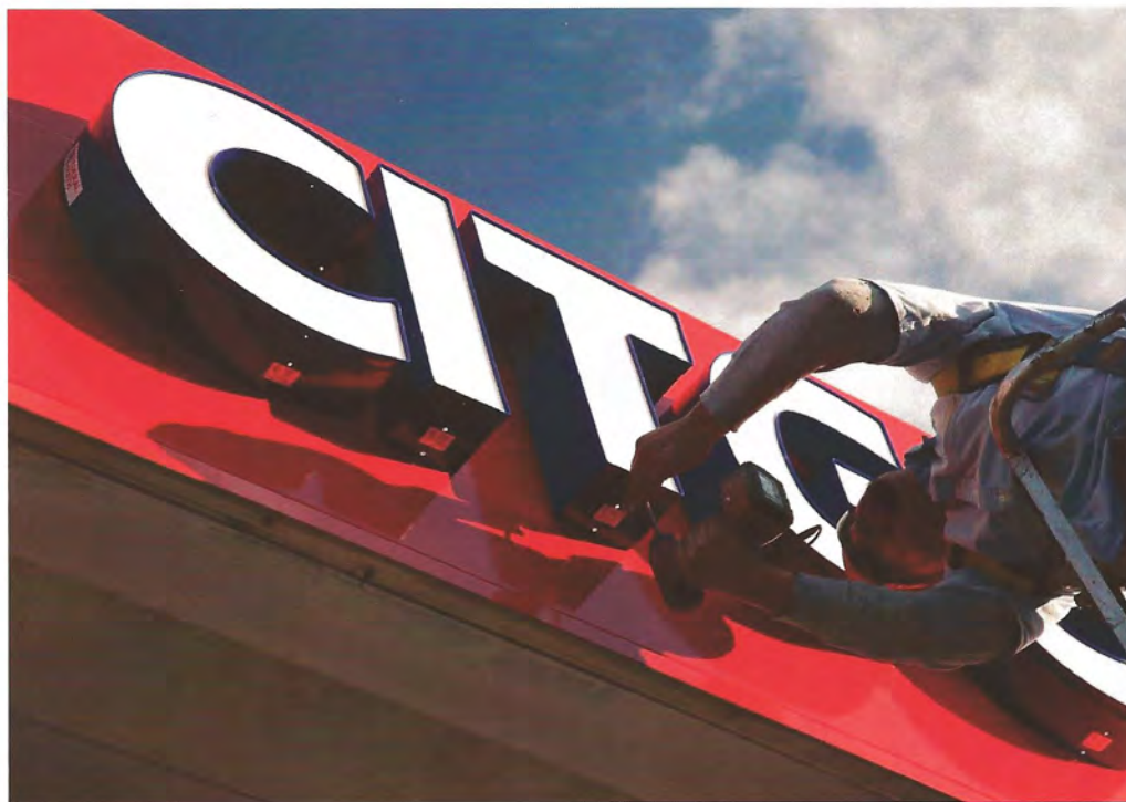
Installing the faces of the white secondary CITGO channel letters. Note that they are flush mounted and the sides of the channel letters are blue.
