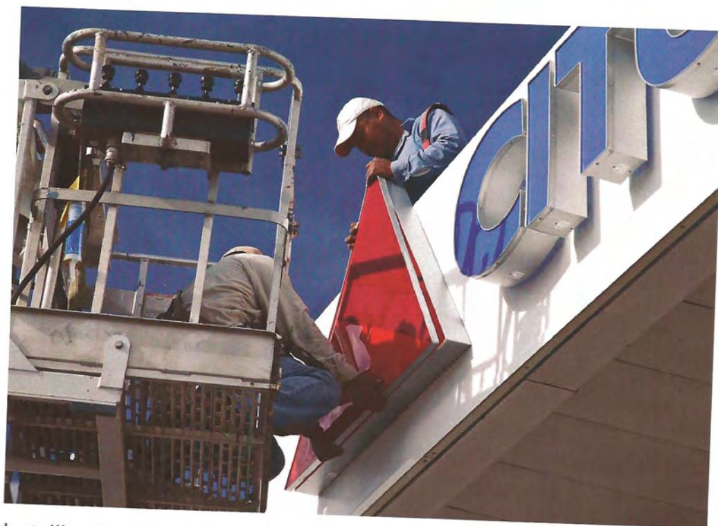
Installing the Trimark and channel letter faces.
