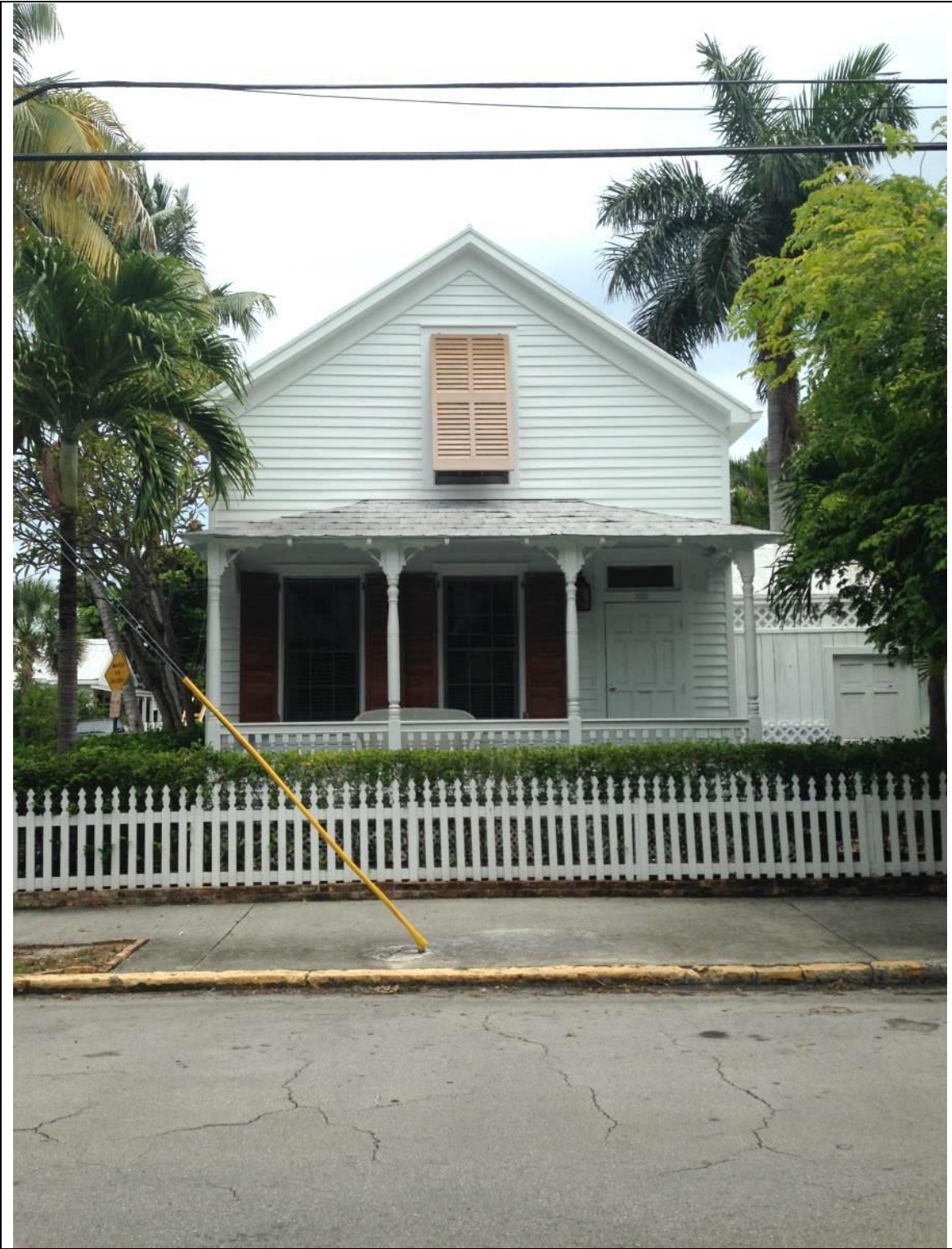
1. 1112 Southard Street. View from the street.
