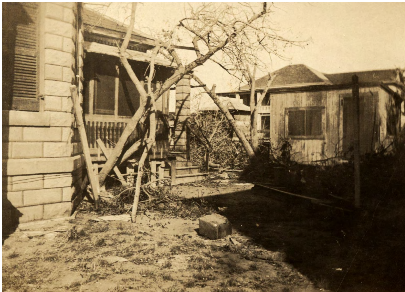
Backyard damage from 1919 hurricane. Monroe County Library.
