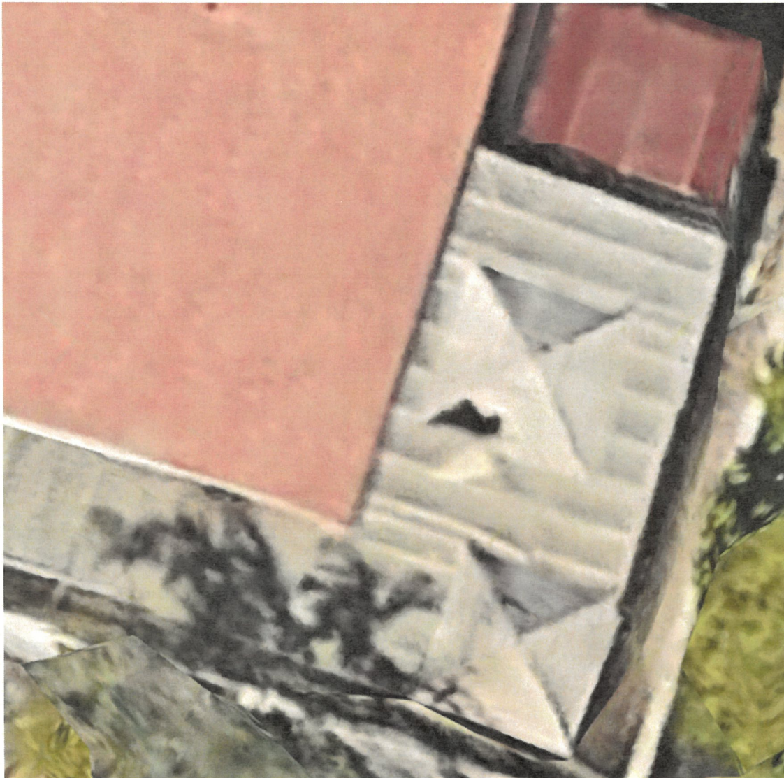
Aerial Photograph from August 19, 2022, showing hole in porch roof
