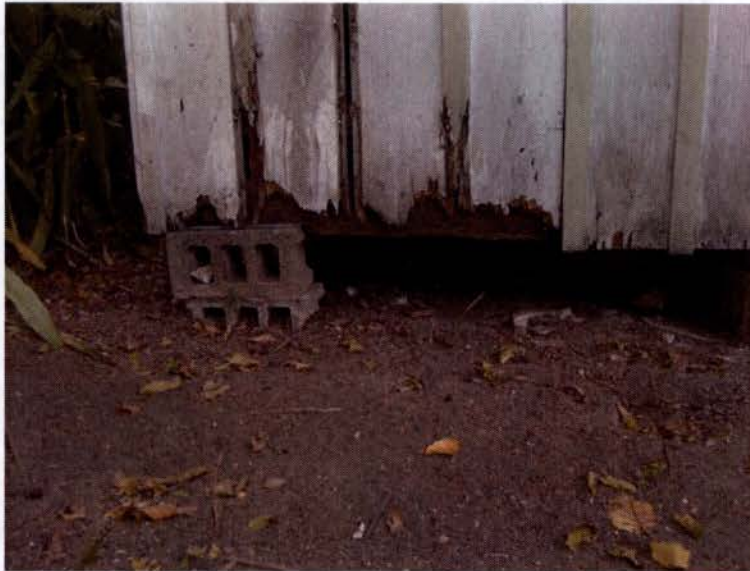
EXISTING BLOCK PIERS TO BE REMOVED AND REPLACED WITH NEW CONCRETE PIERS
