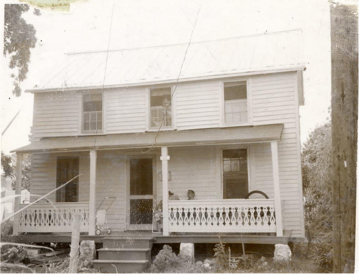
1965 photo showing the main building at 6 Fletchers Lane.
