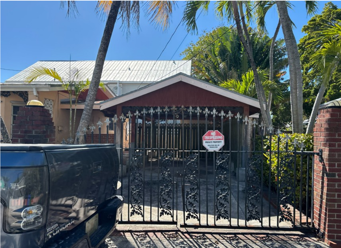
1012 Howe Street Carport and Front gate
