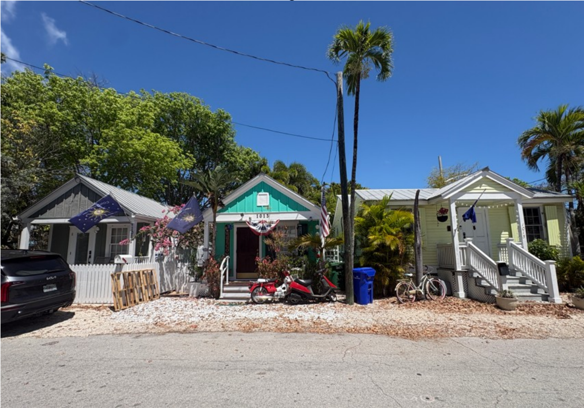
1011, 1013, and 1015 Howe Street – Directly across the street
