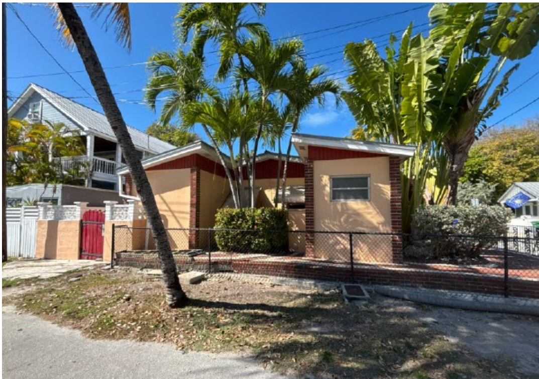
Photo of Property Under Review from Julia Street.
