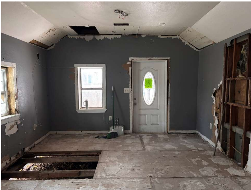
General view of interior. Finishes include Plywood flooring, Gypsum Board Walls and ceilings.
