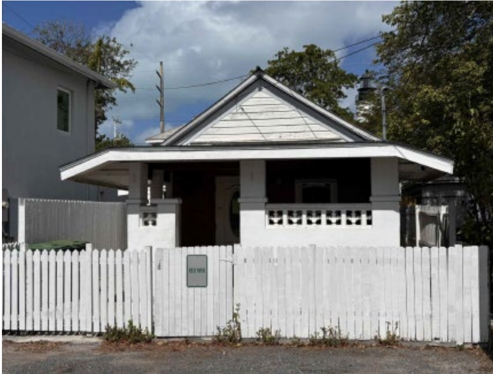
Photo of front of property under review showing non-historic porch configuration.
