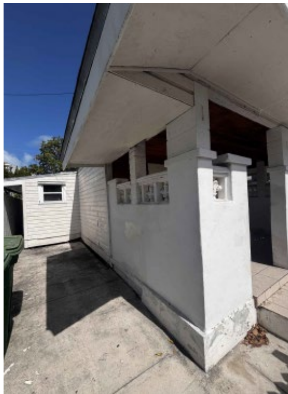
Photo of west side of property under review.
