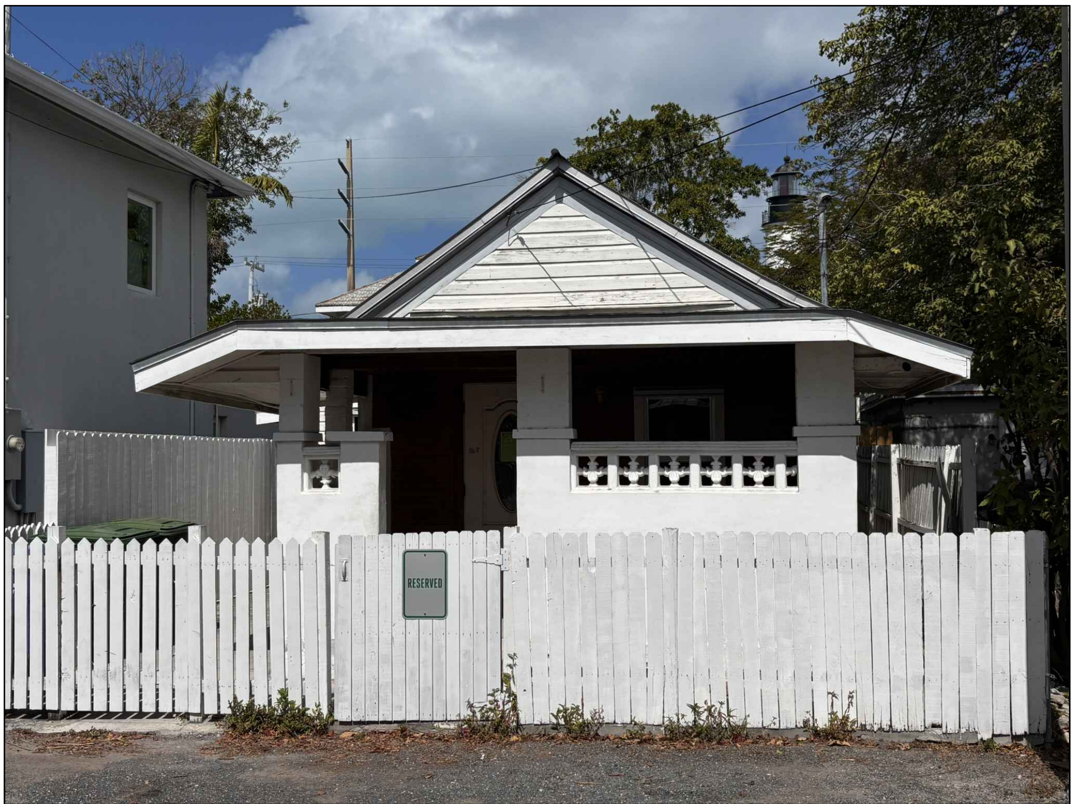
1 A5 PHOTOGRAPH OF THE FRONT OF THE HOUSE (JULIA STREET) N.T.S.
