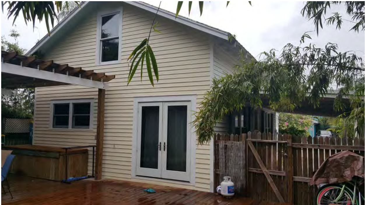
1212 Margaret Street – View from Rear Illustrating Rear Façade
