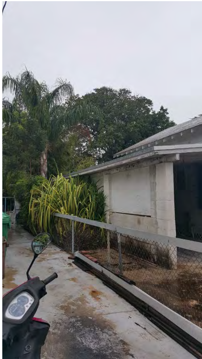
1212 Margaret Street – View from Front Left Illustrating Existing Carport
