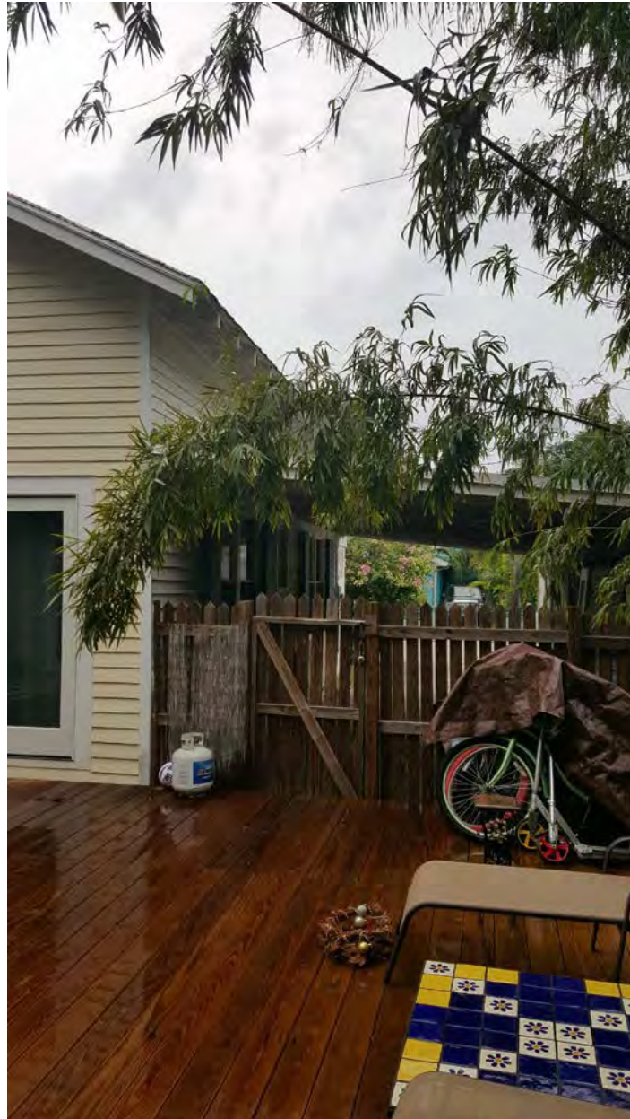
1212 Margaret Street – View from Rear Illustrating Carport
