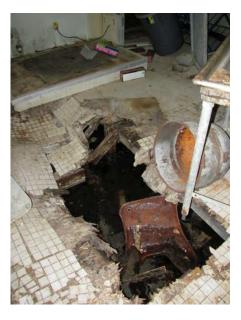
Interior view of the West Cable Hut, showing the collapsed floor. Restaurant equipment has fallen through the plywood floor into the flooded crawlspace below.
