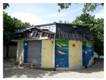
General view of the West Cable Hut. The concrete exterior walls have been covered in murals. Note the large openings cut into the walls for doors. The mansard upper roof structure has been covered with v-crimp roofing, much of which is damaged.
