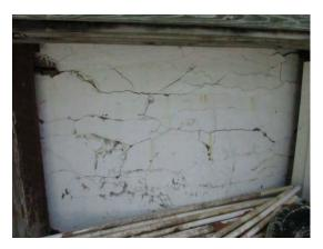
Spalling concrete can be seen at the SW exterior corner of the East Cable Hut.
