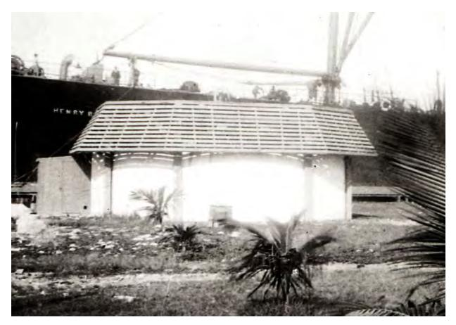
An enlarged version of the previous photo (taken in the 1920's) shows the Cable Hut in detail. The X-Bracing of the wood heavy timber can be seen behind the lattice.
