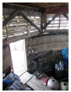
The exterior door can be seen in this interior view of the East Cable Hut. The louvered infill panels can be seen above the door. These panels extend around the entire exterior of the structure.
