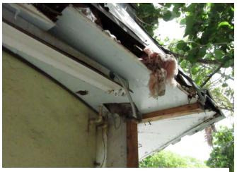
View of the underside of the roof soffit at the West Cable Hut. While the mansard structure is likely historic, it has been heavily altered with the addition of insulation, plywood soffits, wiring, and lighting.
