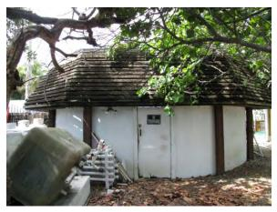
The exterior of the east Cable Hut. The heavy timber columns can be seen spaced around the tank. The door is the only entry into the East Cable Hut.
