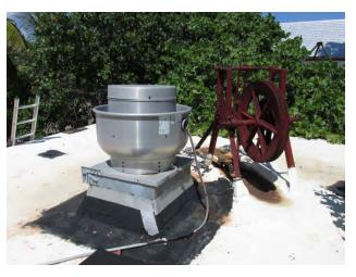
General view of the West Cable Hut roof. The Ansul hood vent is at left and the historic cable winch is at right.
