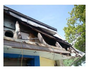
The West Cable Hut mansard roof, showing damaged v-crimp roofing. Parts of the roof framing are original, but have been heavily altered.
