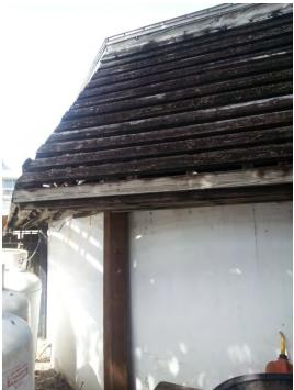
Close-up view of the roof edge of the East Cable Hut. This roof consists of 2x4's gapped 5" o.c. over a 2x wood frame.
