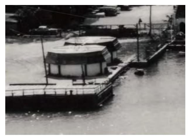
1958 photo of the Cable Huts. The lattice 'mansard' roofs along the sides of the tanks are still intact. The roof hatches are visible at the top. No winches or pulleys can be seen at the roof tops.
