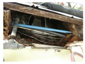
A view of the existing exterior soffit at the West Cable Hut. Several utilities are exposed, including wiring in flexible conduit, gas lines, romex conduit, and what appears to be low voltage wire.
