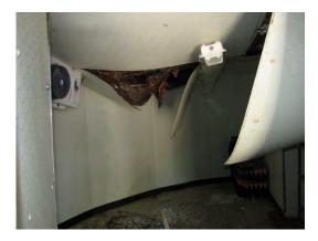
A view of the walk-in refrigerator at the West Cable Hut. The ceiling has collapsed due to leakage.
