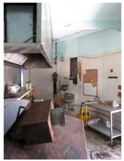
A view of the restaurant kitchen at the West Cable Hut. The pizza oven at foreground has fallen through the rotted floor. Electrical conduit can be seen running along the walls.
