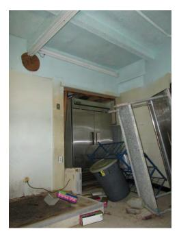
Typical interior view of the West Cable Hut, showing painted gypsum board ceilings, FRP walls, and Vinyl flooring. Note decayed restaurant equipment.
