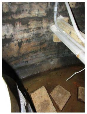
The original concrete wall and floor of the East Cable Hut can be seen in this photo. The concrete floor of the tank lies approximately 36" below grade, and is flooded with approximately 3" of water.
