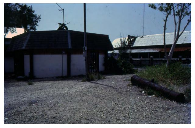
This photo of the Cable Huts was taken in 1984. This is a photo of the west cable hut, looking south. A wood shingle roof has been added to the original wood lattice roof of the structure. The cable winch can be seen on the roof of the building. This winch is still there today.
