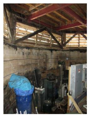
The interior of the East Cable hut. The concrete tank wall can be seen at bottom. The heavy timber structure is above the tank wall. Wood louvers have been installed between the top of the concrete tank and the roof. Note steel beams spanning the roof.
