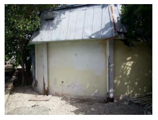
The exterior of the West Cable Hut, showing the 6" x 8" heavy timber columns ringing the tank. The columns are deteriorated at their bases, but otherwise appear in good condition.
