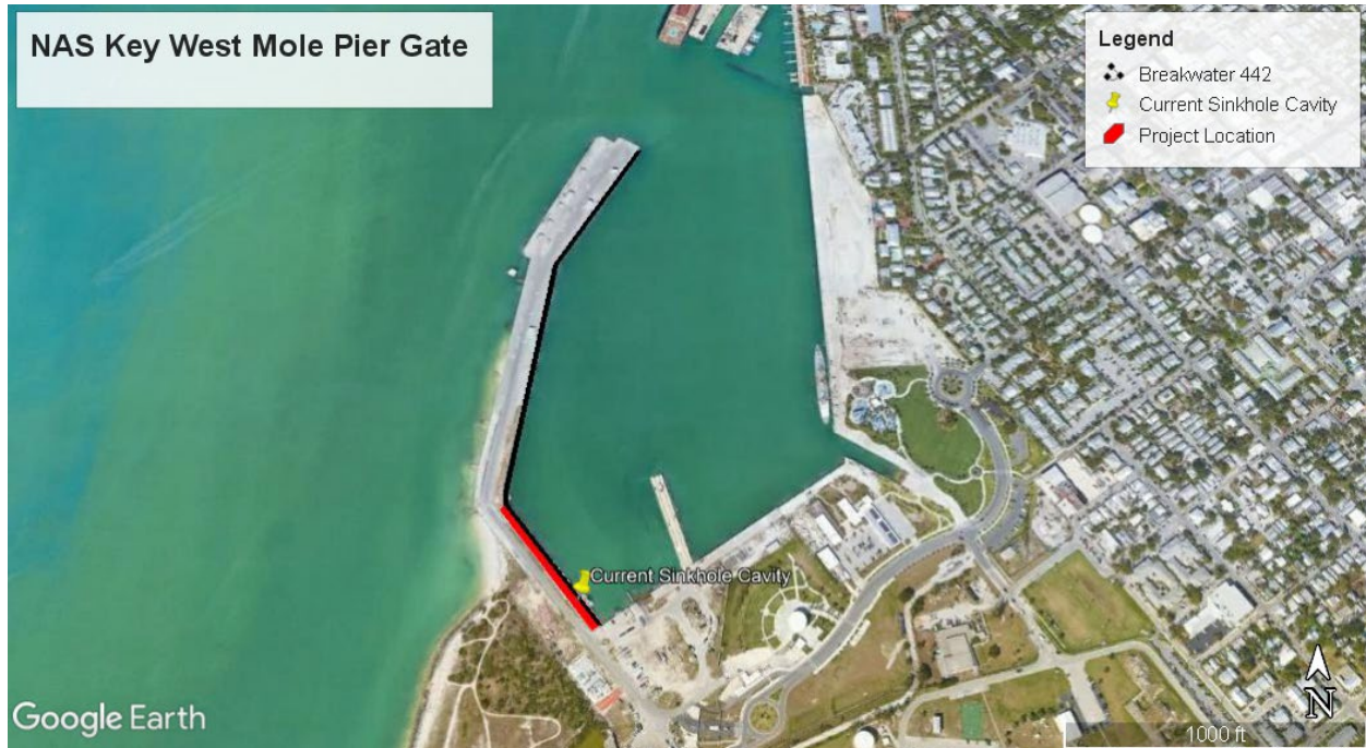
Insert 1: Location of Project Limits (Red Line) along NAS Key West Mole Pier.
