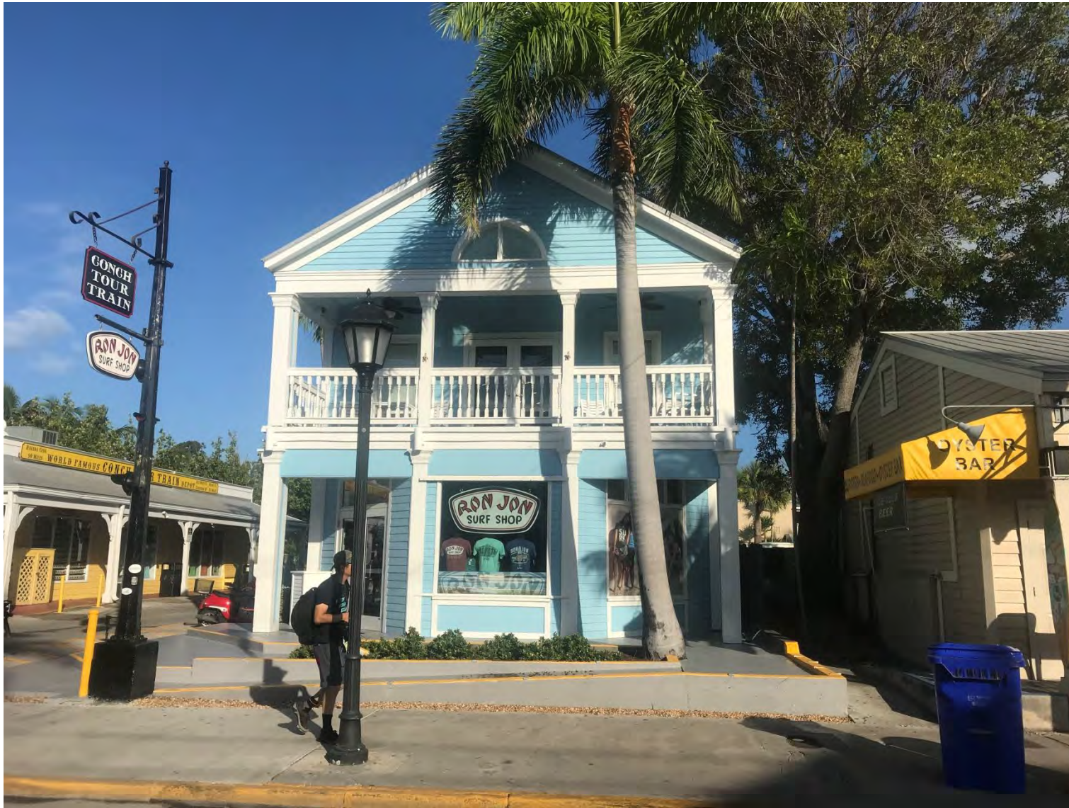
503 FRONT STREET RIGHT NEIGHBORING PROPERTY FRONT VIEW
