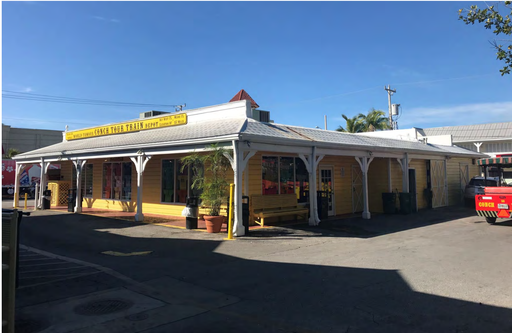
501 FRONT STREET SIDE REAR VIEW
