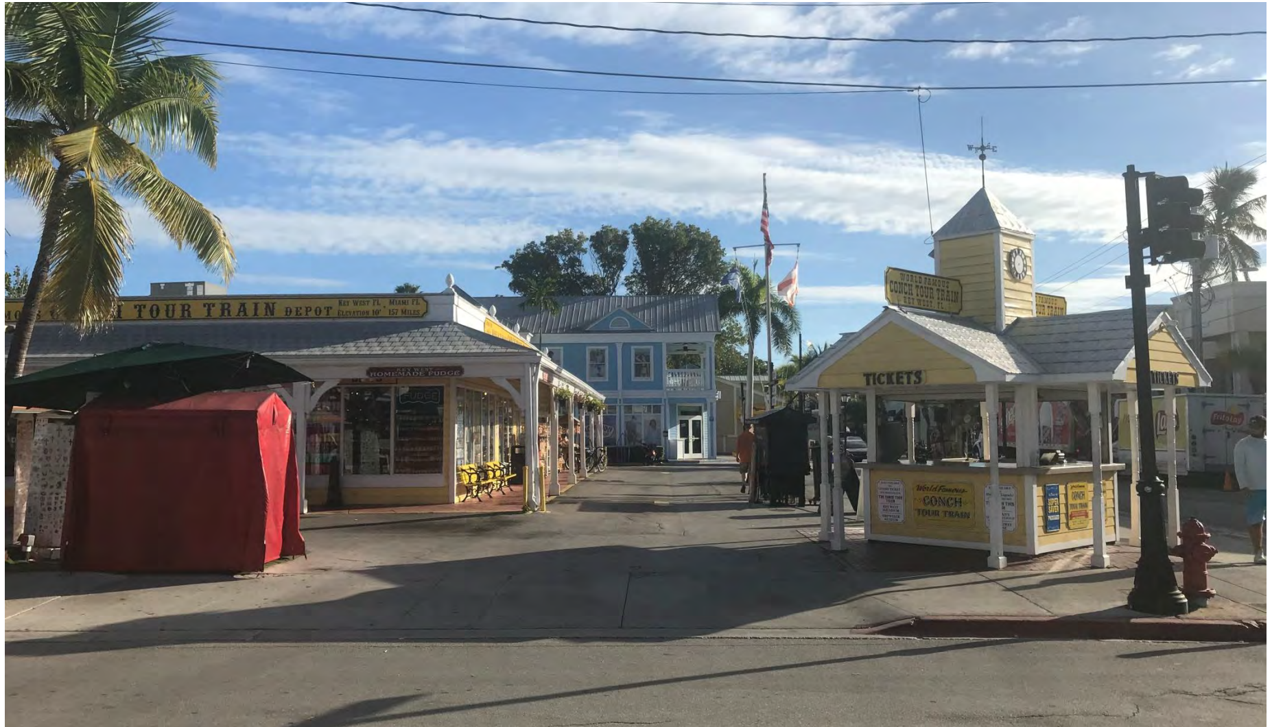
501 FRONT STREET SIDE VIEW
