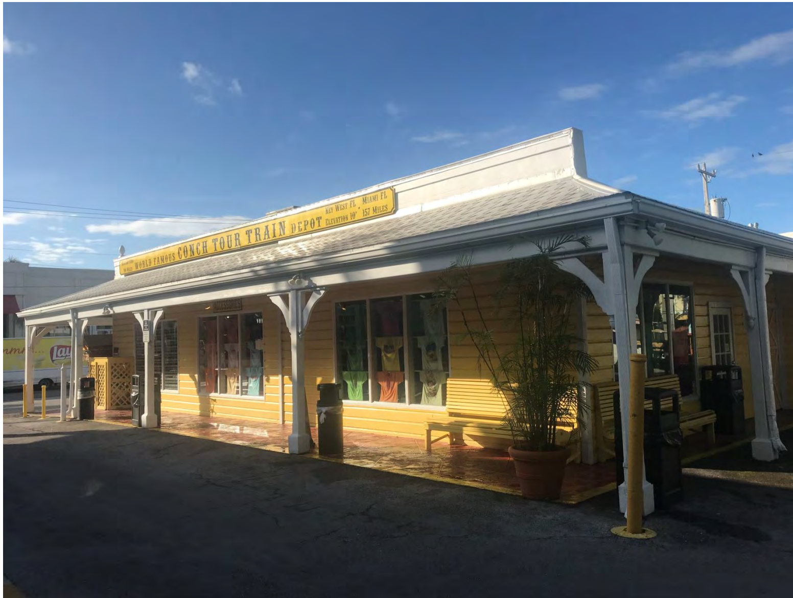
501 FRONT STREET SIDE VIEW
