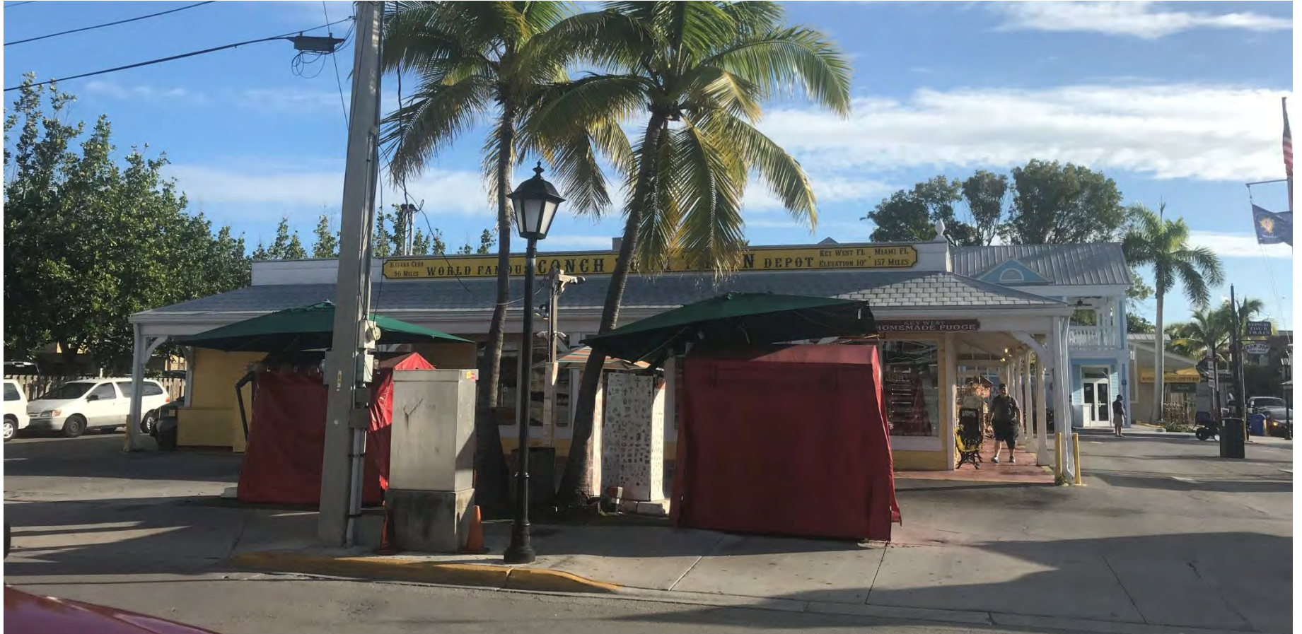
501 FRONT STREET SIDE VIEW
