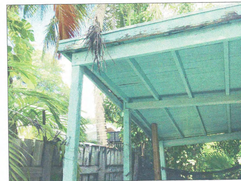
FIGURE 6 VIEW OF PORCH ROOF
