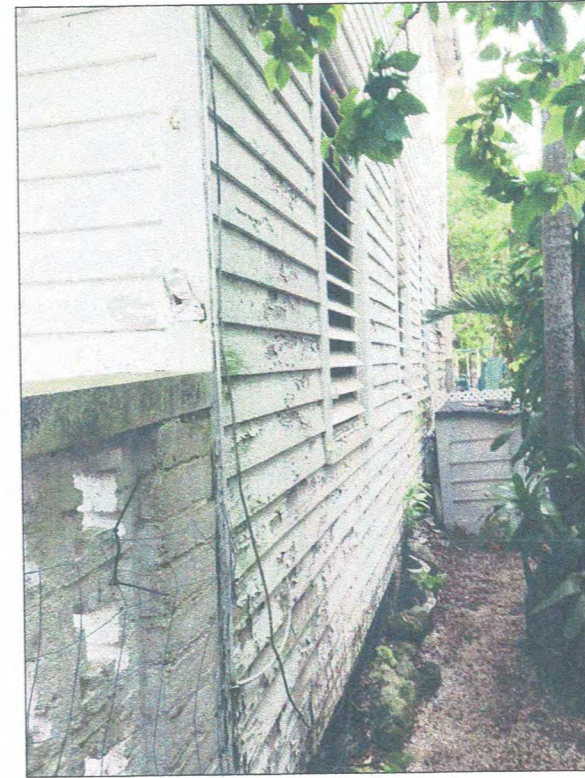
FIGURE 3 RIGHT VIEW OF HOUSE
