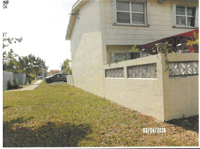
Standing at the northeast project corner looking down the eastern project area.
