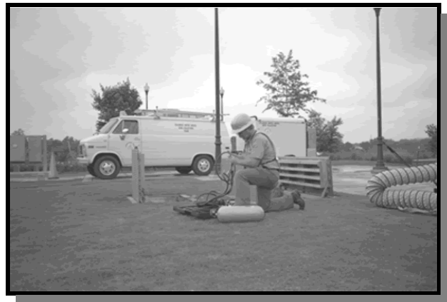
A sewer inspection is an important part of a sewer system capacity evaluation (photo: N.J. Department of Environmental Protection).
