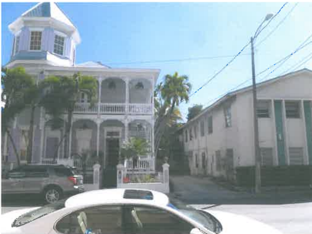
Adjacent Property (534 Eaton St.)
