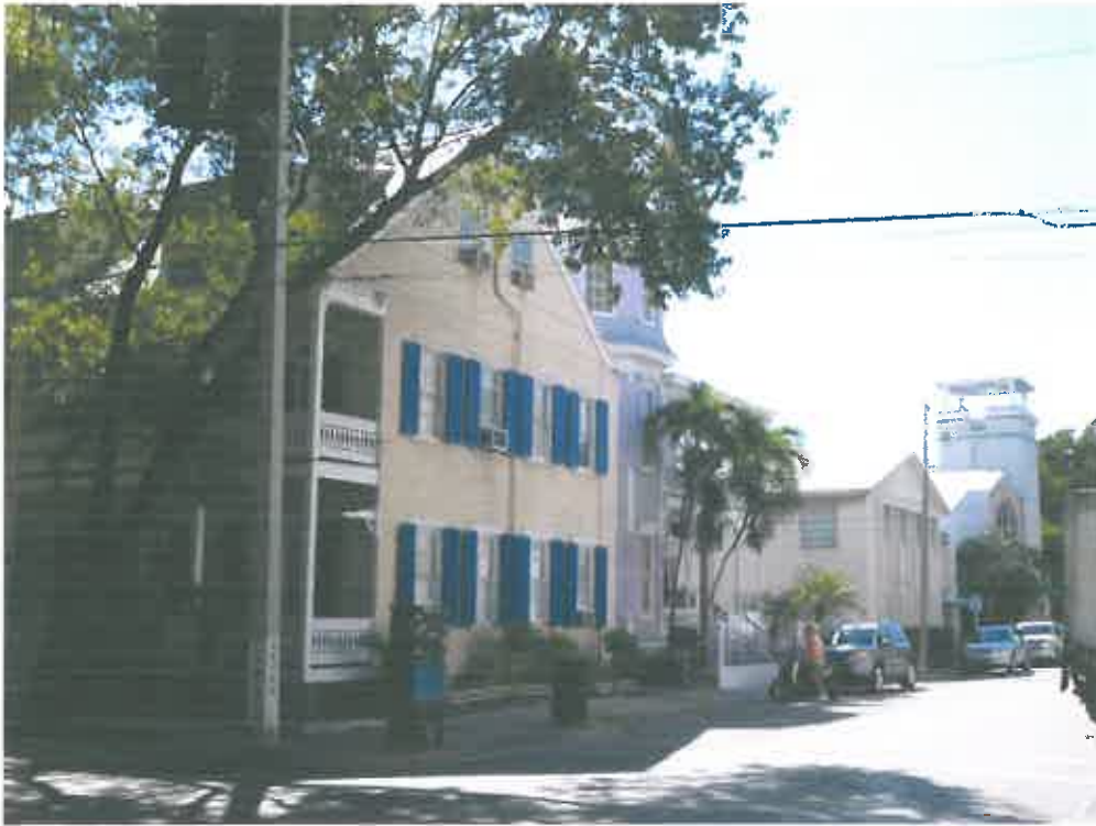
View down Eaton Street (from across Simonton St.) towards site
