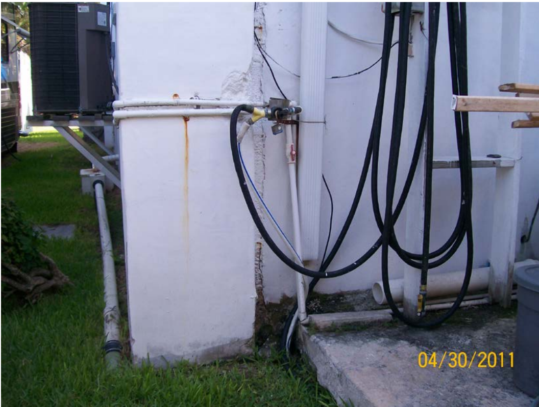
RV #6 - leading from rv to main building.
