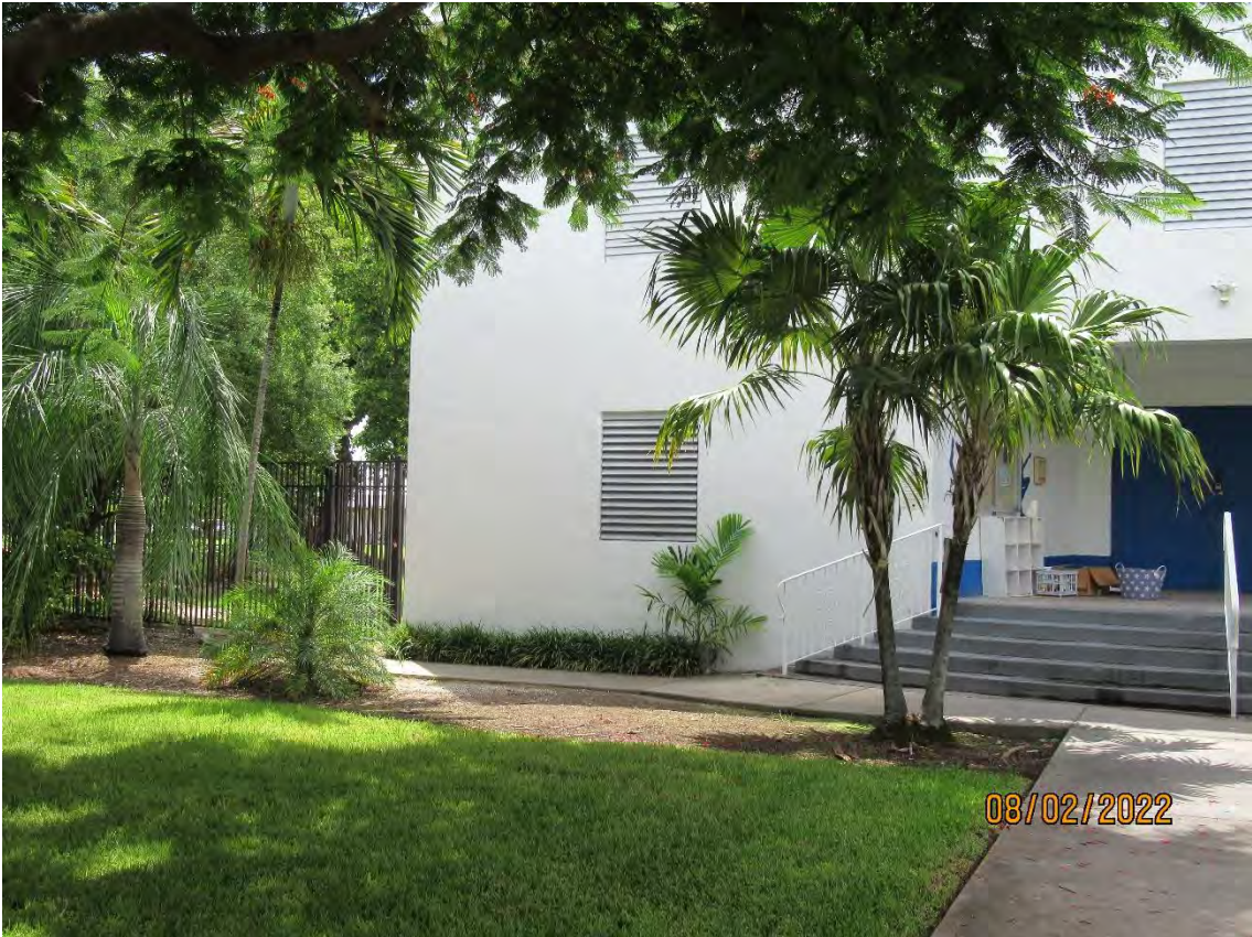
Front of the proposed work area, location of trees # 26-28. All existing trees to be protected from construction impacts.
