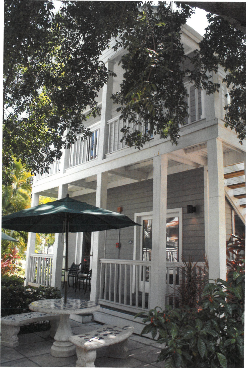
East - Before Construction (opposite Elizabeth Street)
