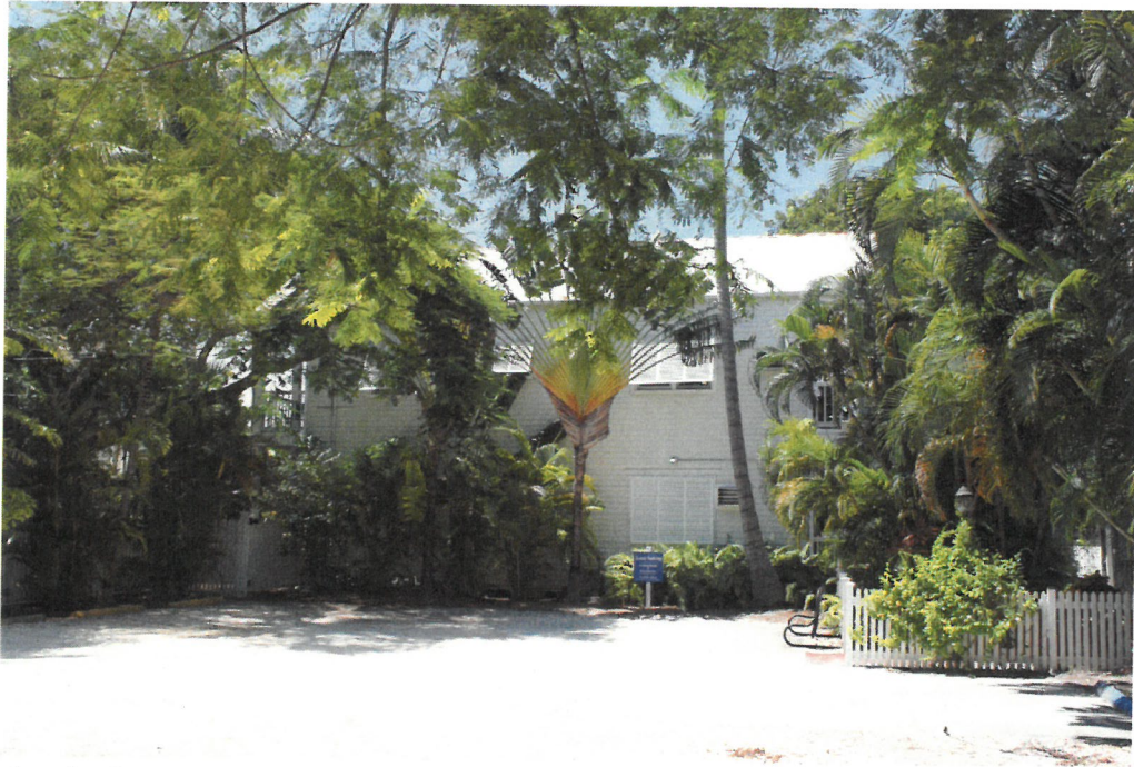
South - Truman Ave View Before Construction
