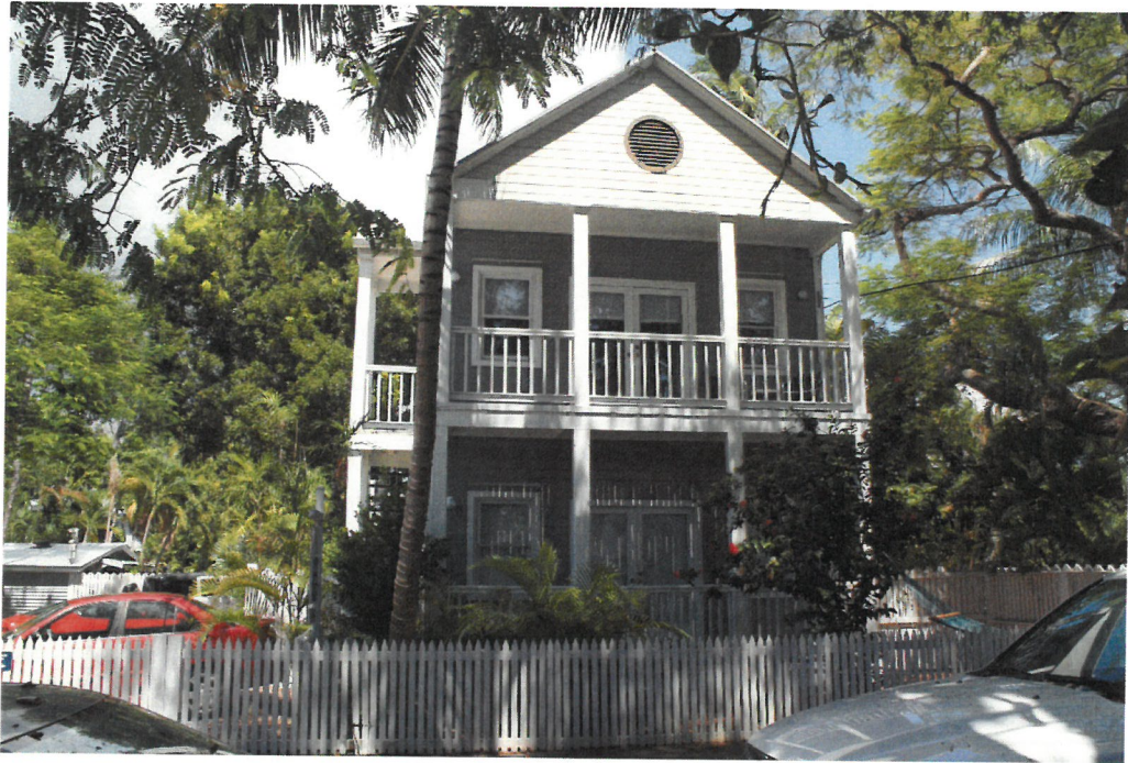
West - Before Construction
