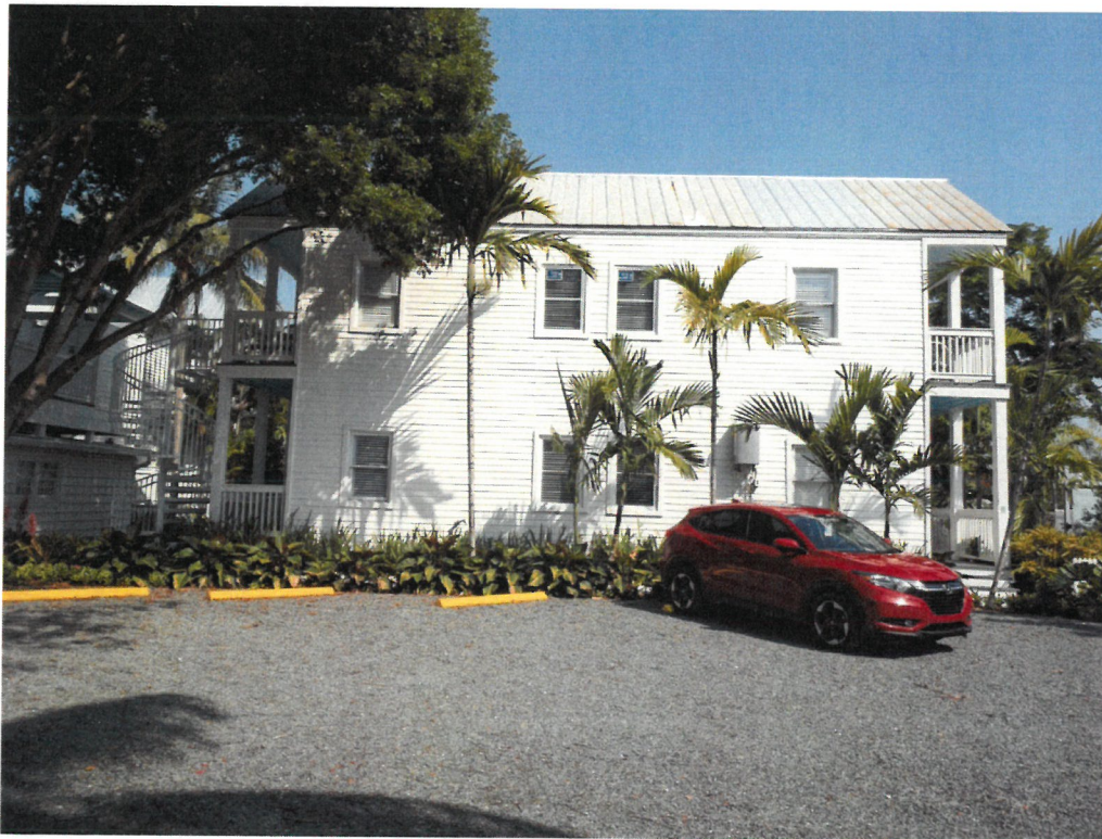
North - Rear View (opposite Truman Ave)
