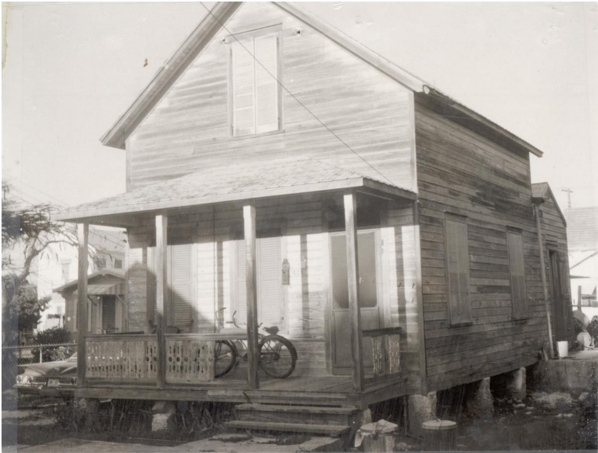
Figure 1 Subject Site: Historic Structure, circa 1965 (Source: Monroe County Library)
