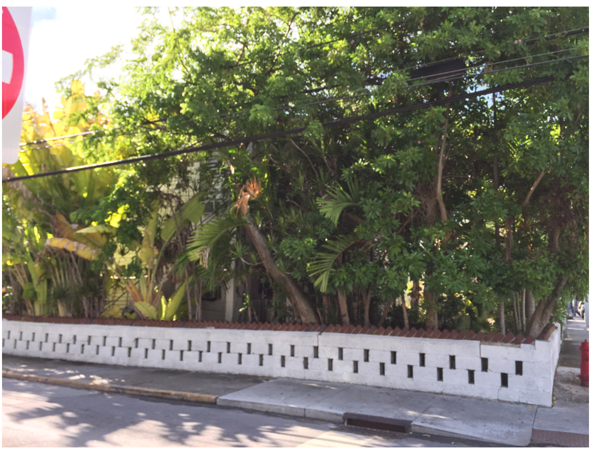
COOPER RESIDENCE - 828 ELIZABETH STREET (OLIVIA STREET SIDE)
