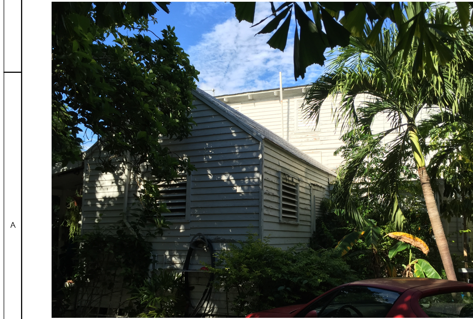
PARTIAL VIEW OF COOPER RESIDENCE FROM OLIVIA STREET / REAR OF PROPERTY
