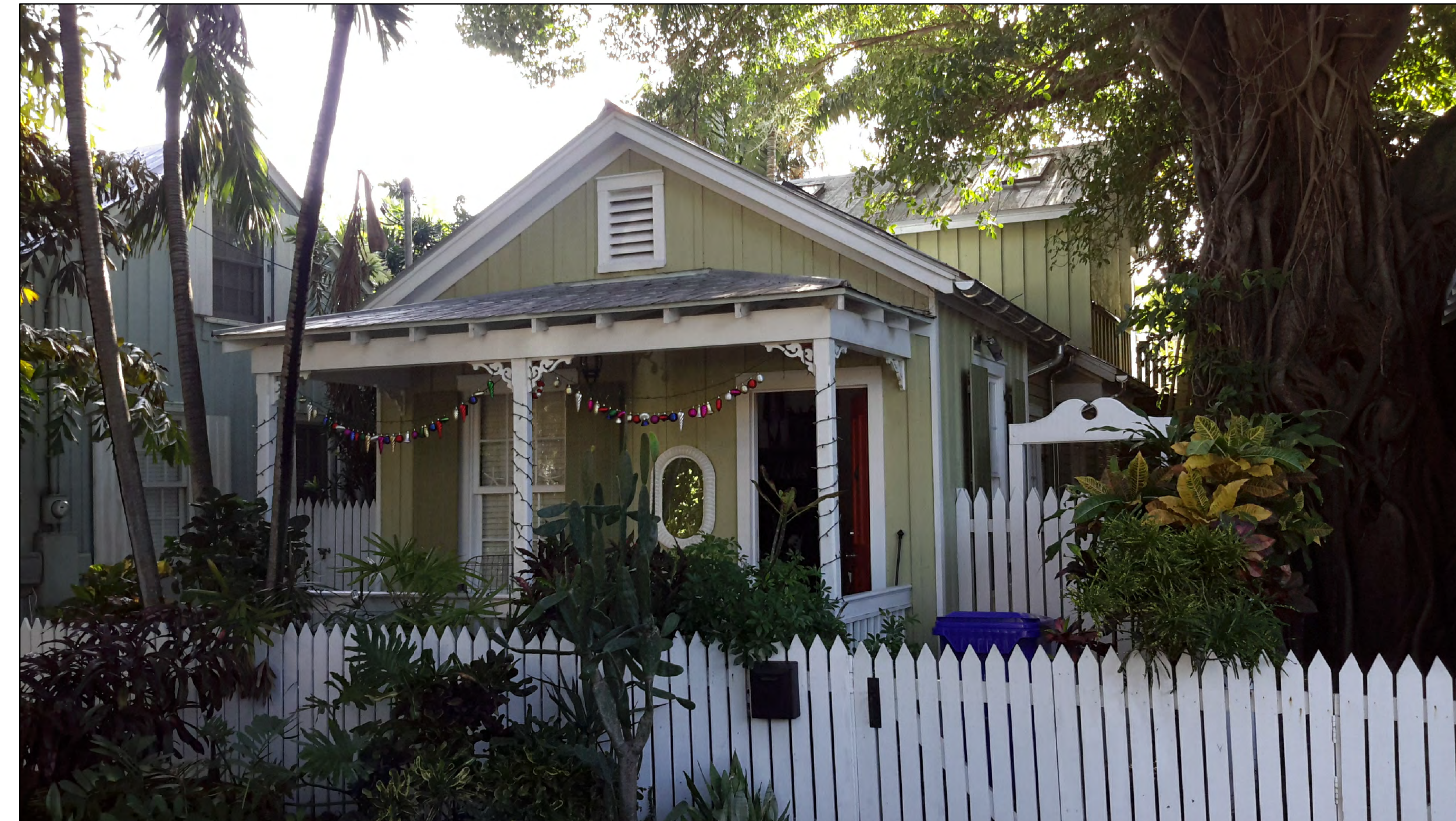
VIEW FROM CARSTON LN.
