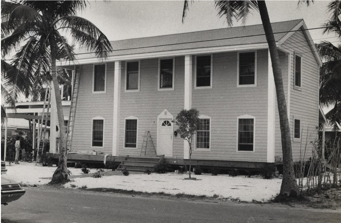
House in 1979 while roof deck was under construction. Monroe County Library.
