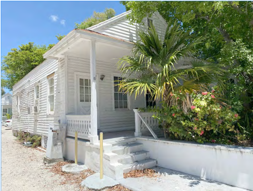
HISTORICAL BUILDING FRONT SIDE VIEW
