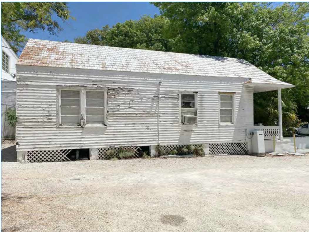
HISTORICAL BUILDING LEFT SIDE VIEW
