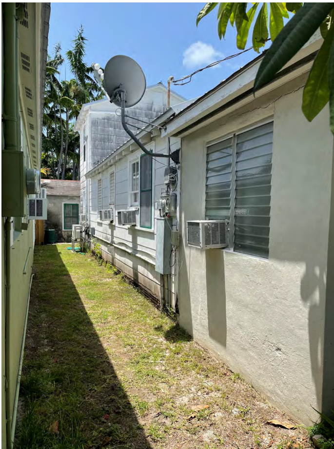
Existing Left Side of House – 1108 Grinnell
