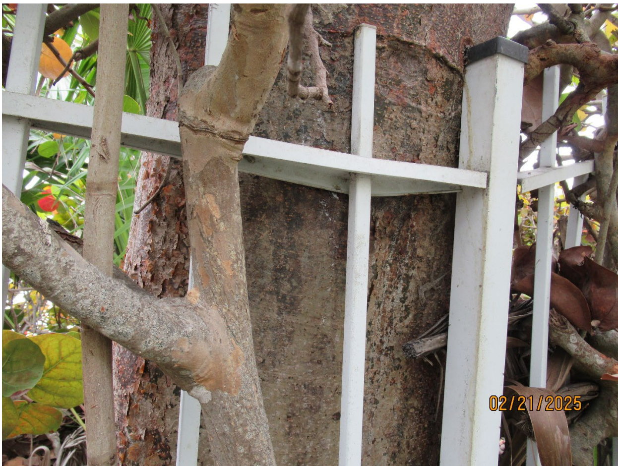
Photos of the fence breaking due to the tree
