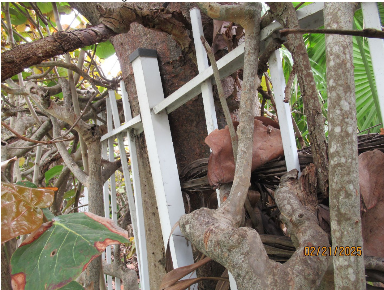
Photos of the fence breaking due to the tree
