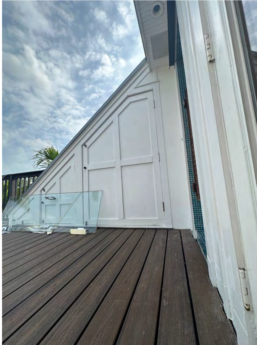
Roof Deck Existing Conditions
