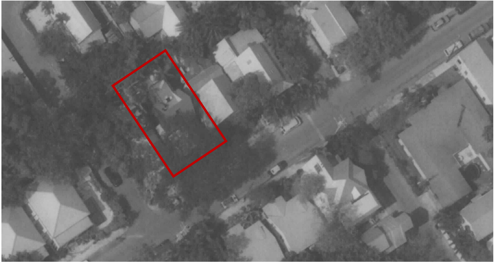
1998 Aerial Altered Two Story Structure at 1217 Newton Street
