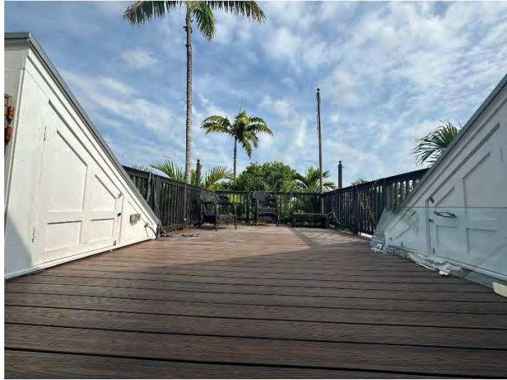
Existing Roof Deck Conditions
