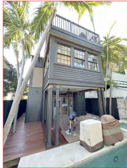
Existing Rear of Historic Structure
