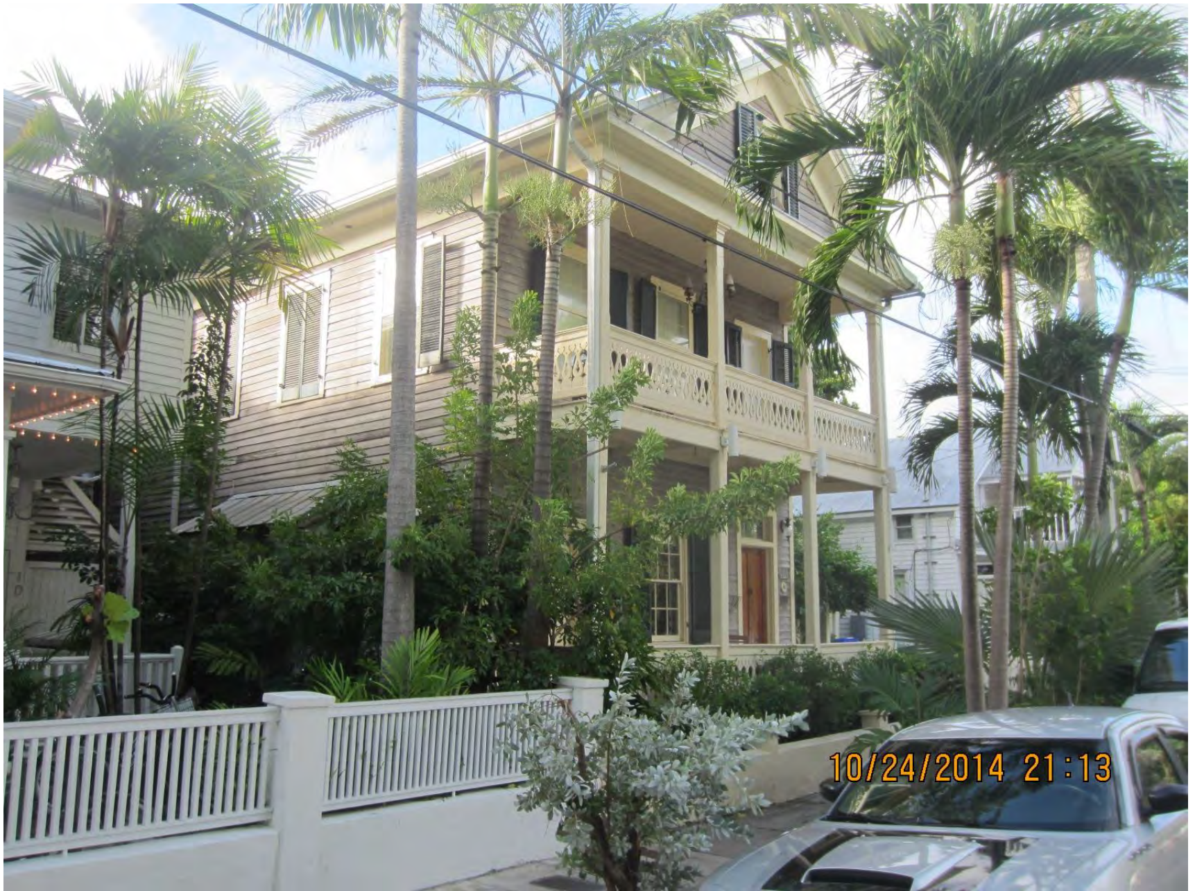
Neighboring Structures on Fleming
