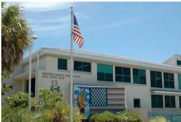
Big Pine Key Fire Station #13
