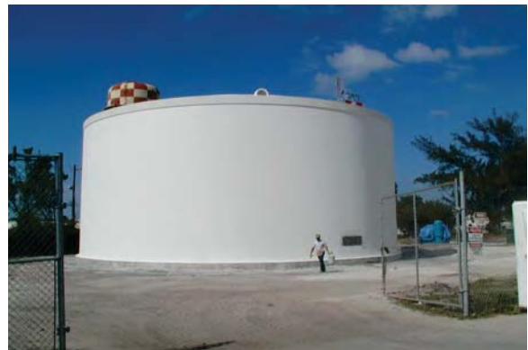
700,000 Gallon Concrete Water Tank
