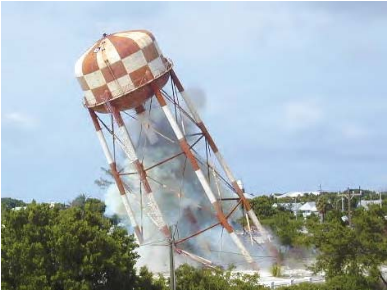
Water Tank Demolition, NAS Key West
