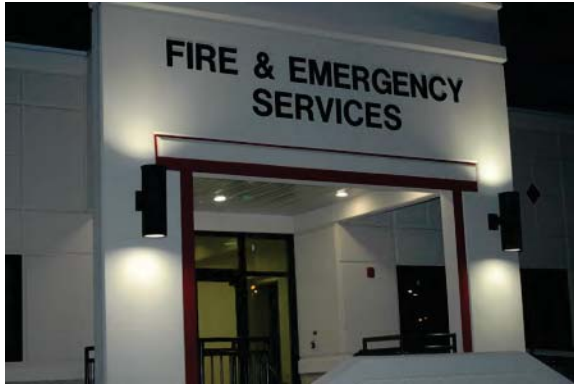
P678 Aircraft Fire & Rescue HQ, Boca Chica NAS
