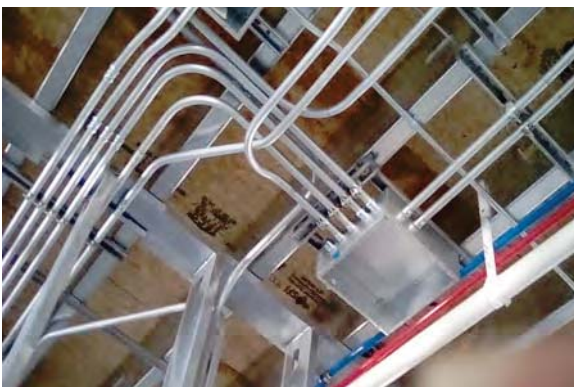
Marathon Utility & Maintenance Building
