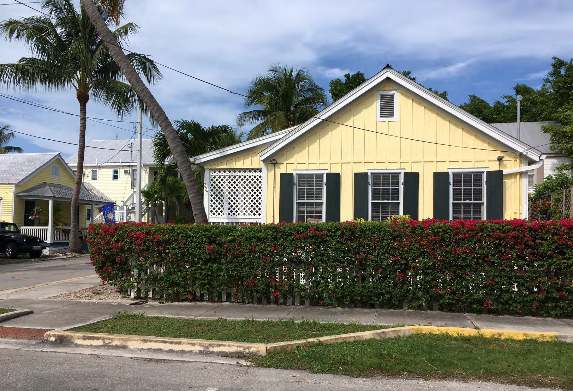
New construction on 227 Virginia Street.
