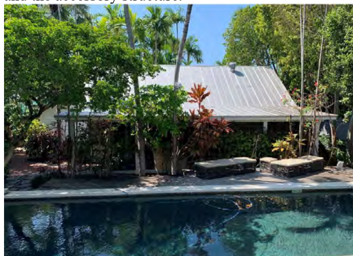
The accessory structure under review, existing.
