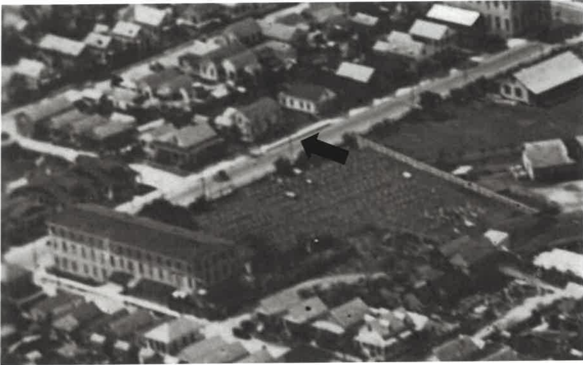
Circa 1920 aerial photo showing 624 White Street. (Key West Public Libraries via Flickr)
