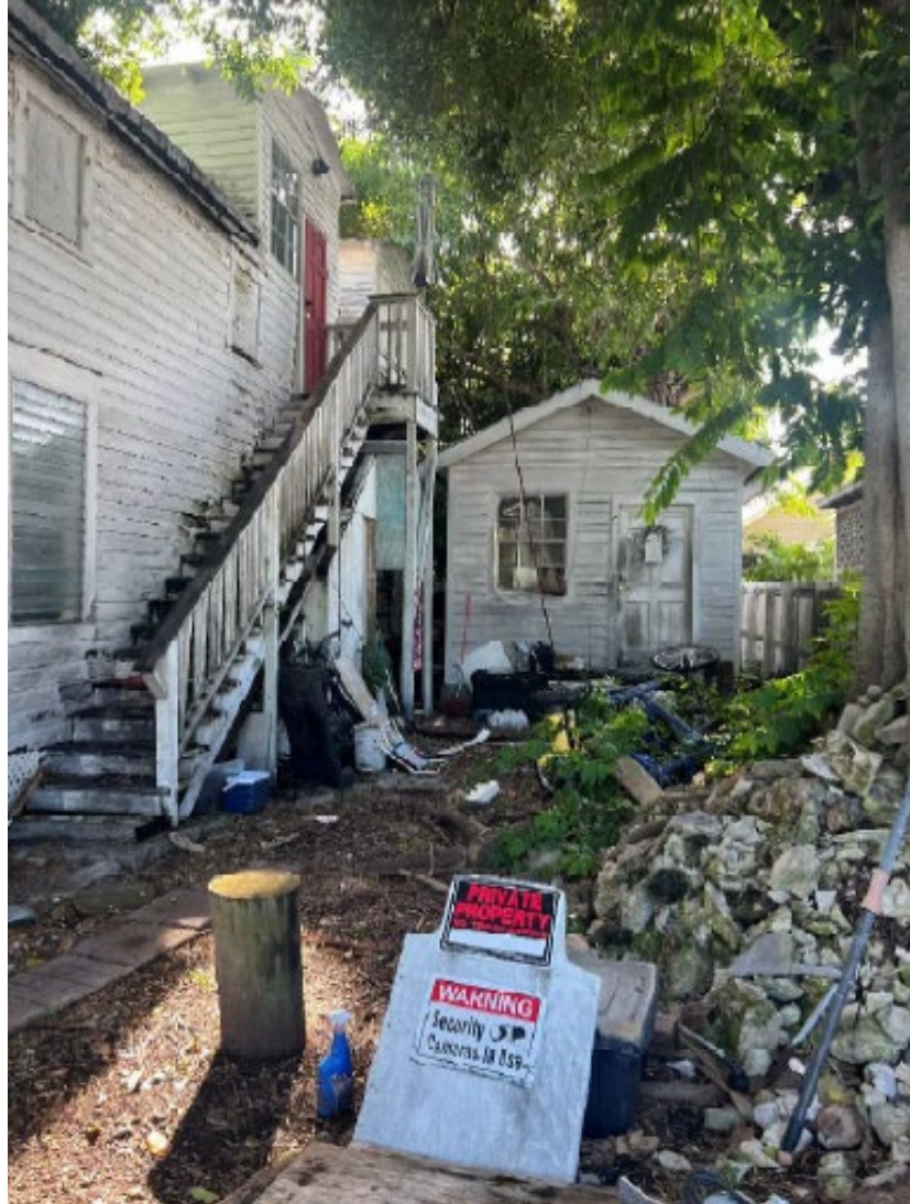
Front view of current accessory structure proposed to be demolished.
