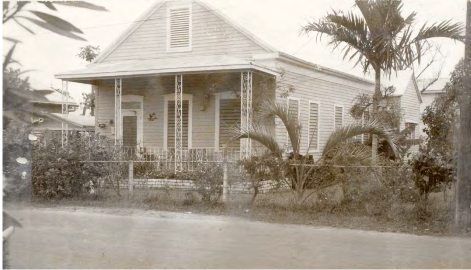
Front and street side elevations circa 1965.
