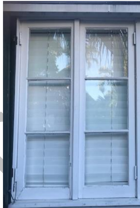
Casement true divide-lite wood window
