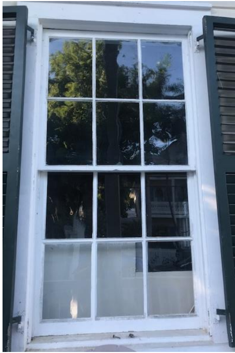
Double-Hung true divided-lite wood window
