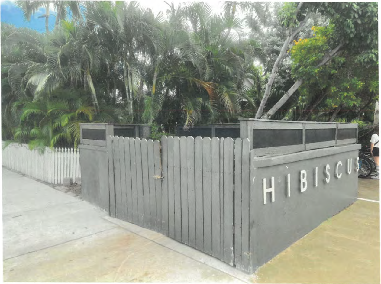
Hibiscus Hotel Dumpster Enclosure directly adjacent to west
