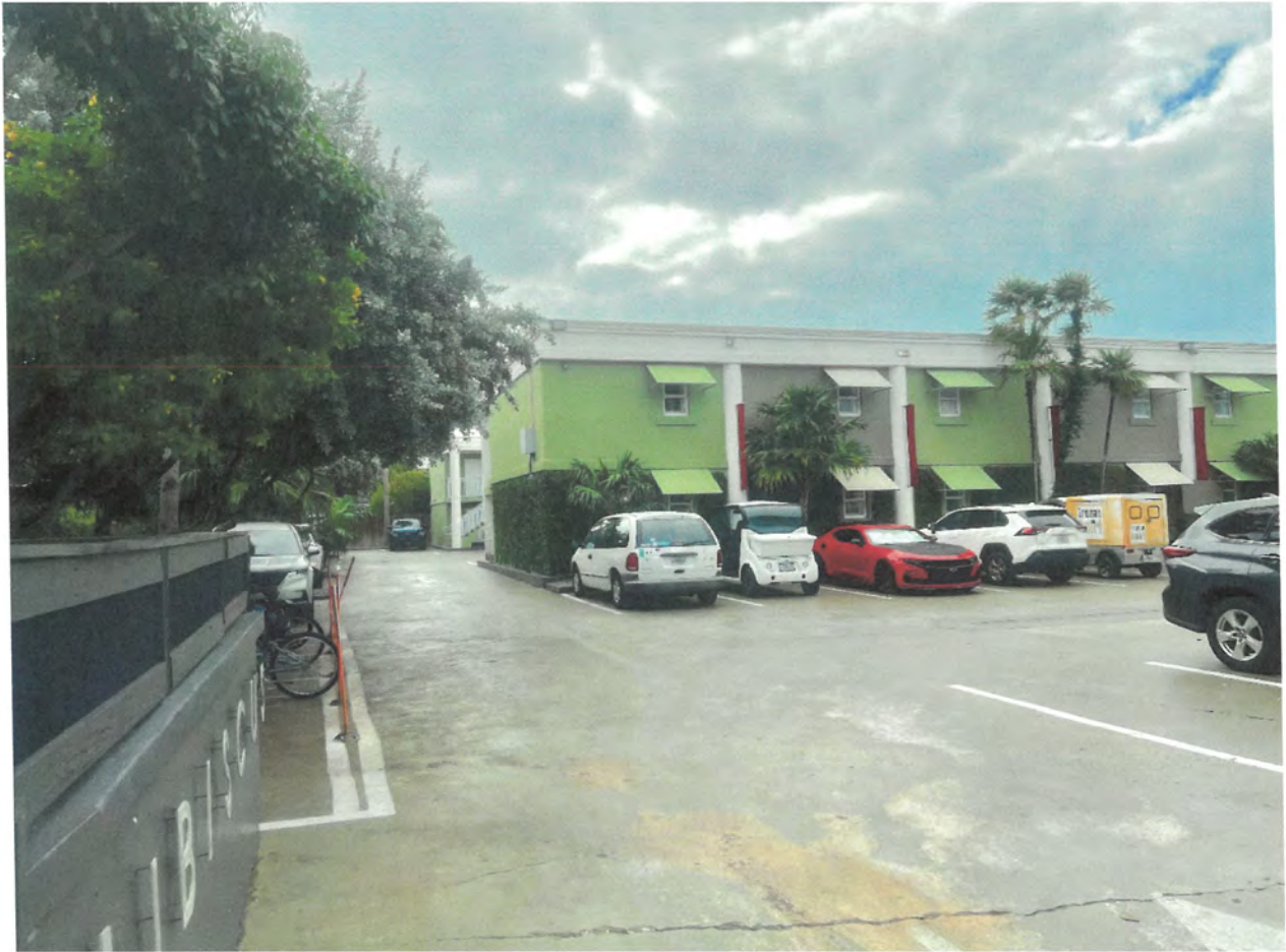
Hibiscus Hotel, dumpster enclosure and parking lot adjacent property to west
