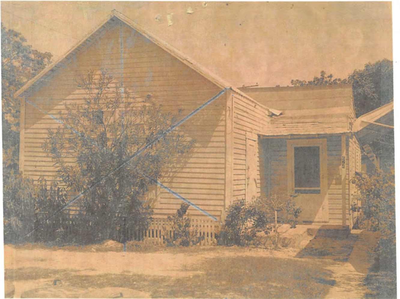
624 United – Historic Photo before demolition of front part of house
