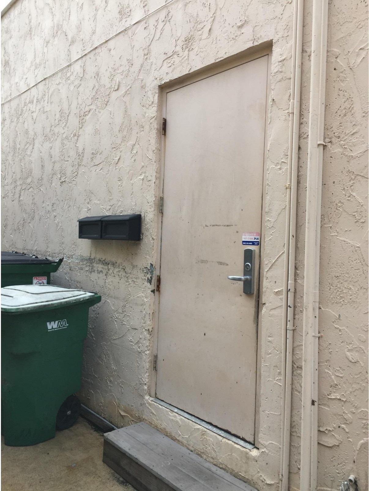
524 Front - street side entrance to second level
