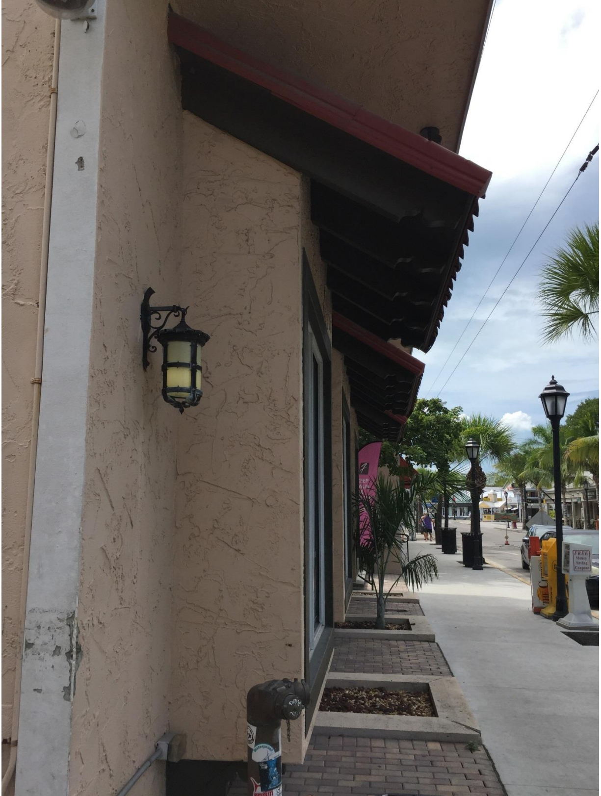
524 Front Street – Front façade showing the existing Spanish style awning
