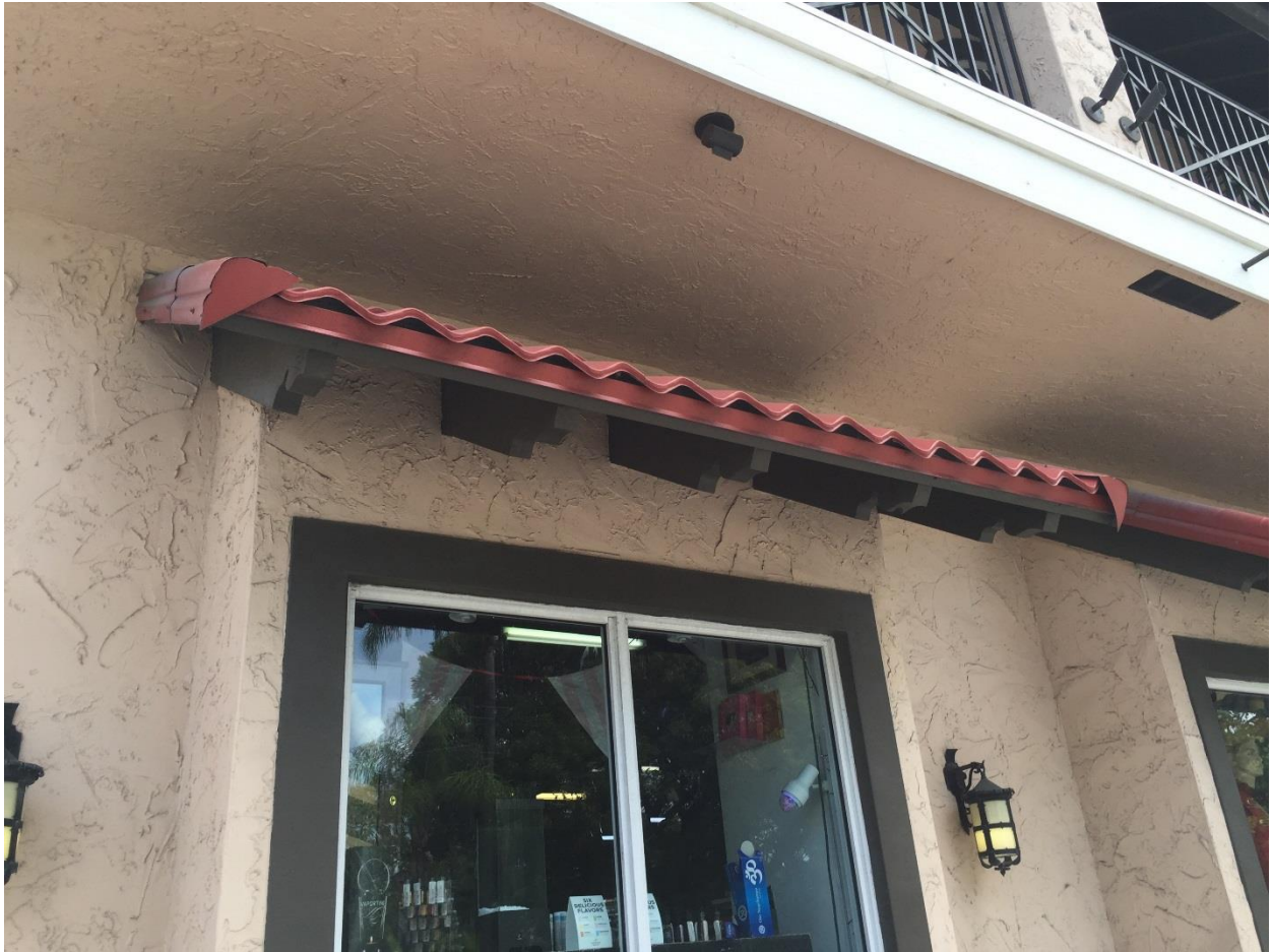
524 Front Street – awning and second level
