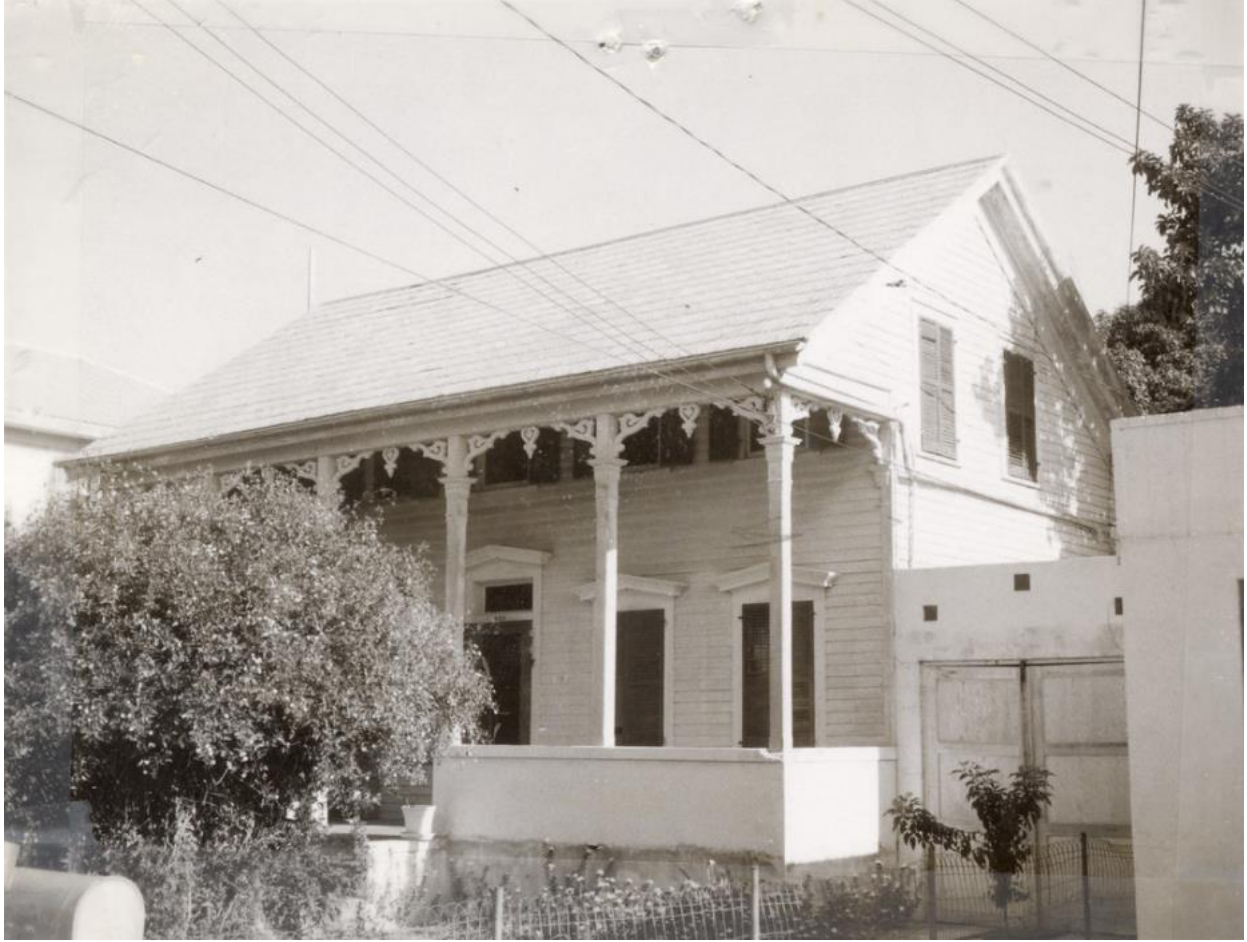
1965 photo of the house at 643 William Street.
