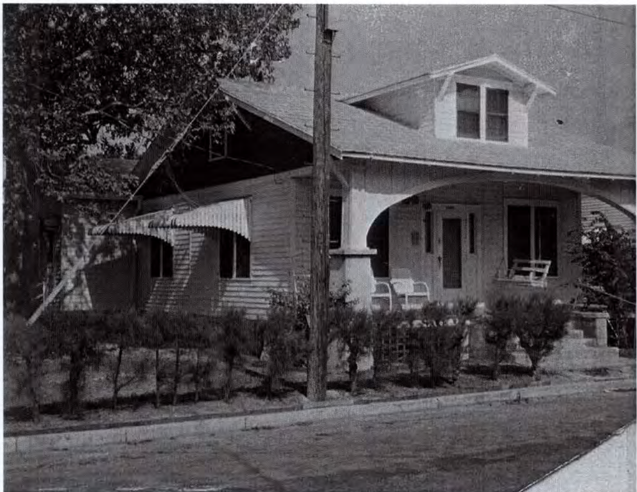
Photo taken by the Property Appraiser's office c1965; 1207 Pine St.; built c1912; Monroe County Library
