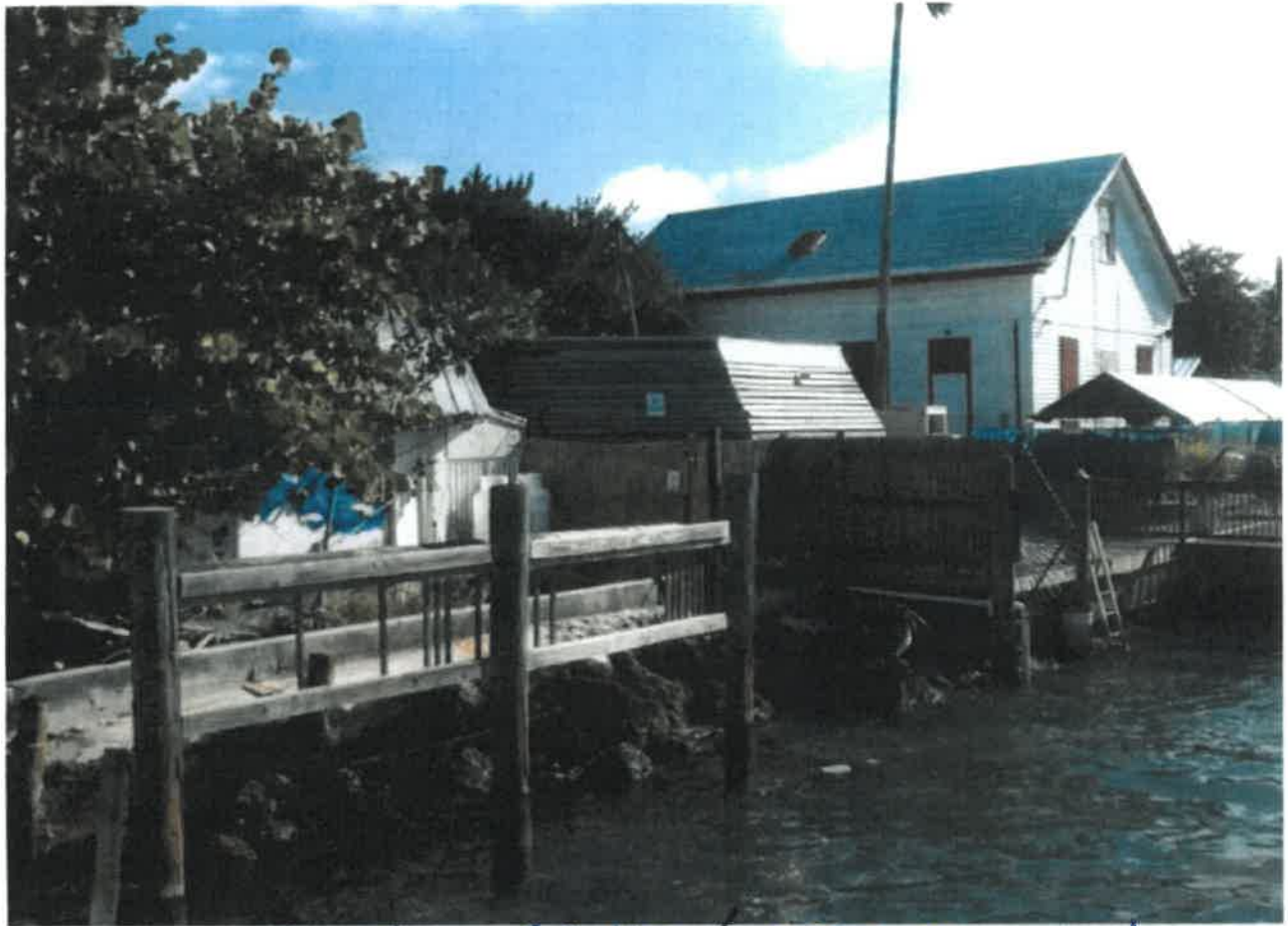
EXISTING BROKEN/ROTTED DECK BEHIND CISTERN
