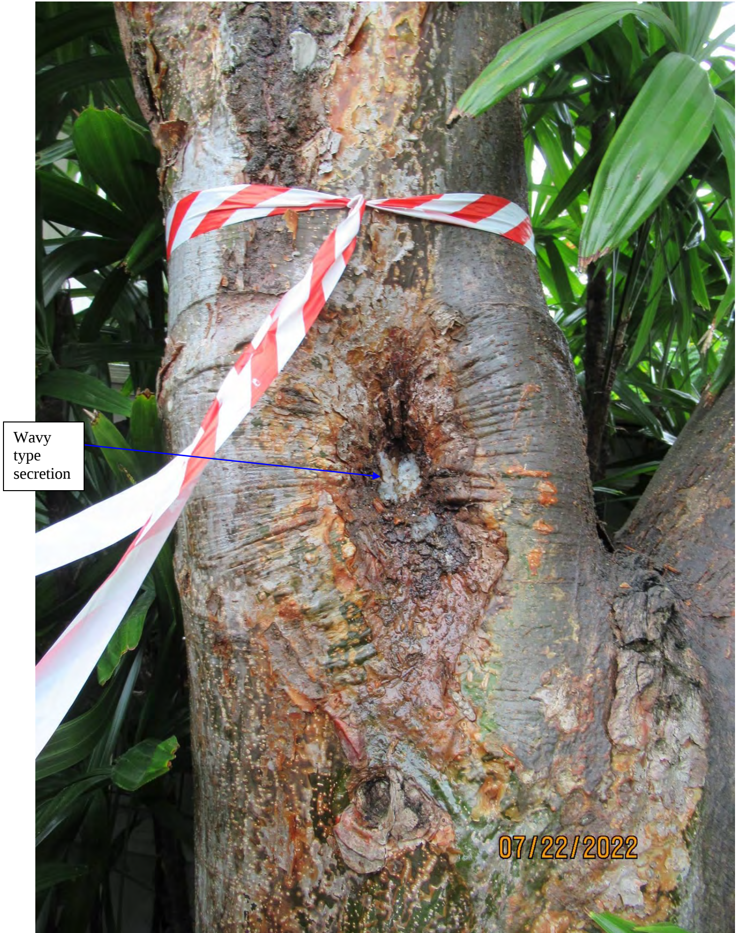
Photo of old injury/damaged area, view 4.
