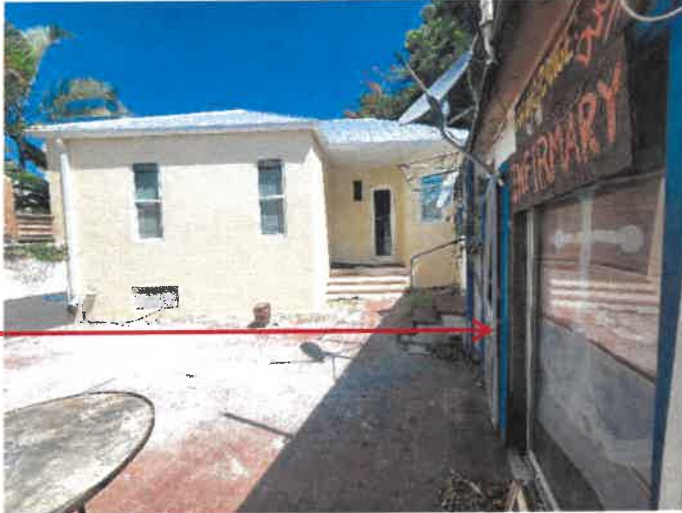
Showing where new structure was built. Condemned building to the right.
