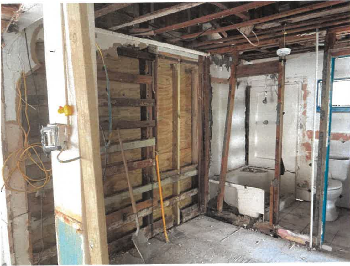
Photograph 2: Interior of the structure.
