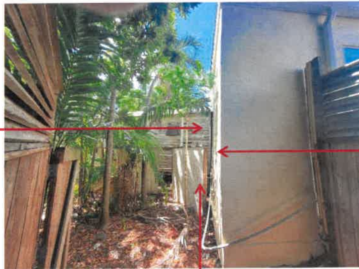
Condemned structure to the left of new structure. There is a small gap between the properties.
