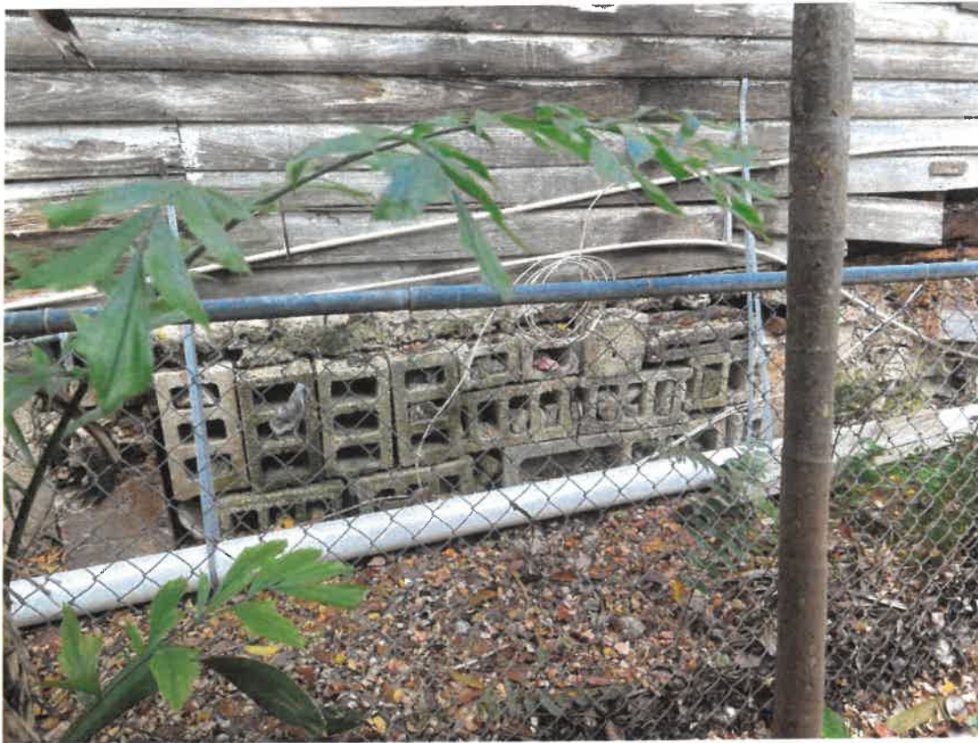
Photograph 6: Another photograph showing the foundation. .
