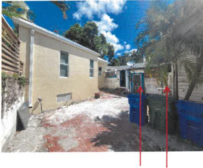
Side view where new structure was built
