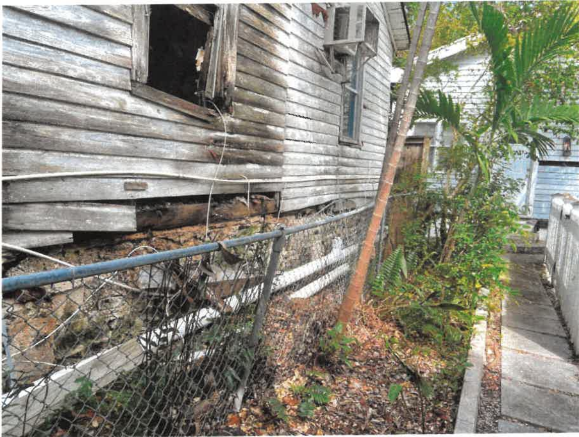
Photograph 4: Photograph of the exterior showing the damaged siding, rim beam and deteriorated foundation.
