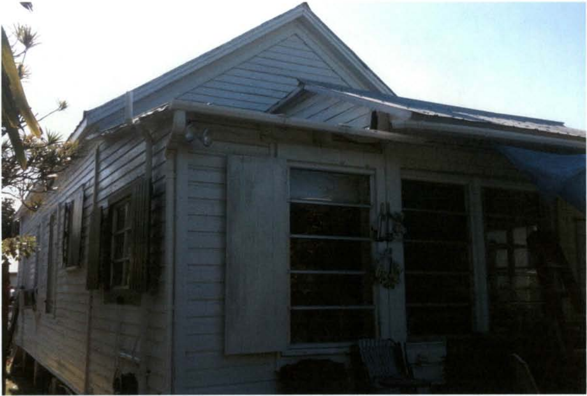
REAR NON-HISTORIC ADDITION
