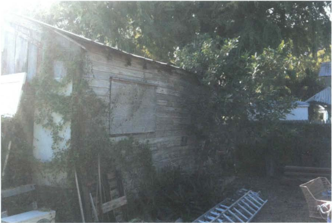
REAR YARD SHED
