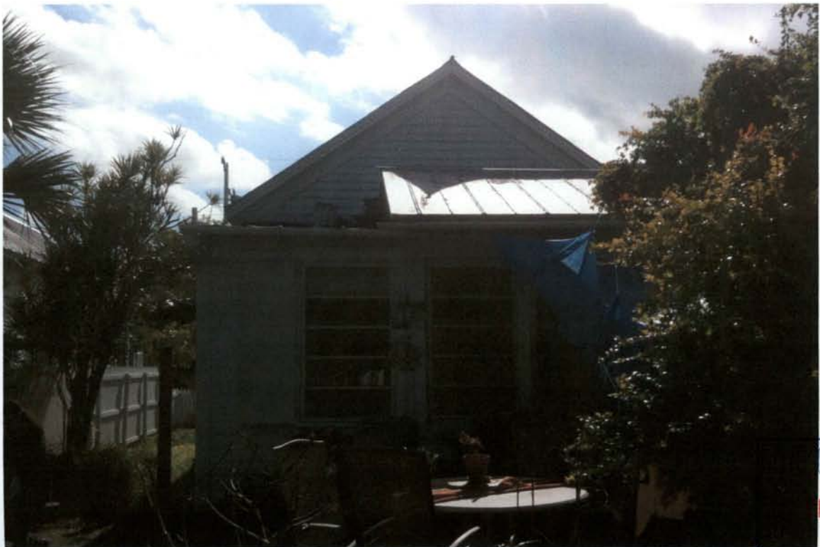
REAR FACADE OF MAIN HOUSE w/ NON-HISTORICAL ADDITION
