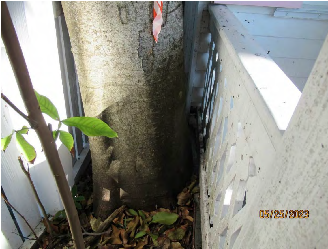
Close up photo of base of tree and foundation of structure.
