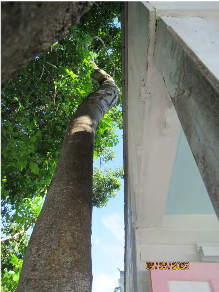
Photo of tree trunk in relation to structure.
