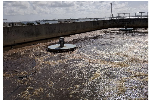
Figure 4-7. Scum Trapped from the Aerobic to Pre-anoxic Zone Backflow Induced by Airlift
