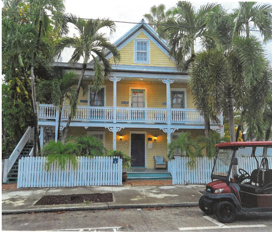
Photo of Front of Property Under Review.
