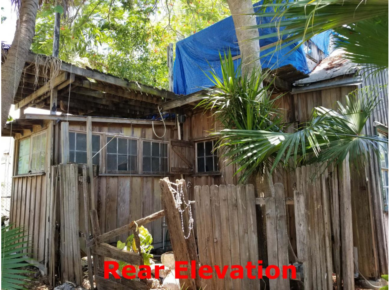
Rear elevation of the structure at 1007 Thomas Street.
