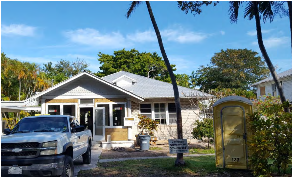
1117 South Street [Behind 1122 Seminary St.]
