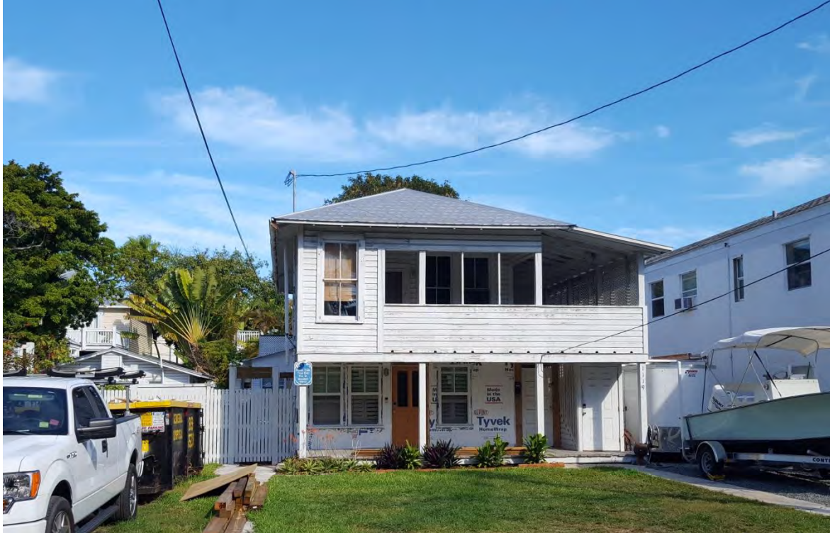
1119 South Street [Behind 1124 Seminary St.]
