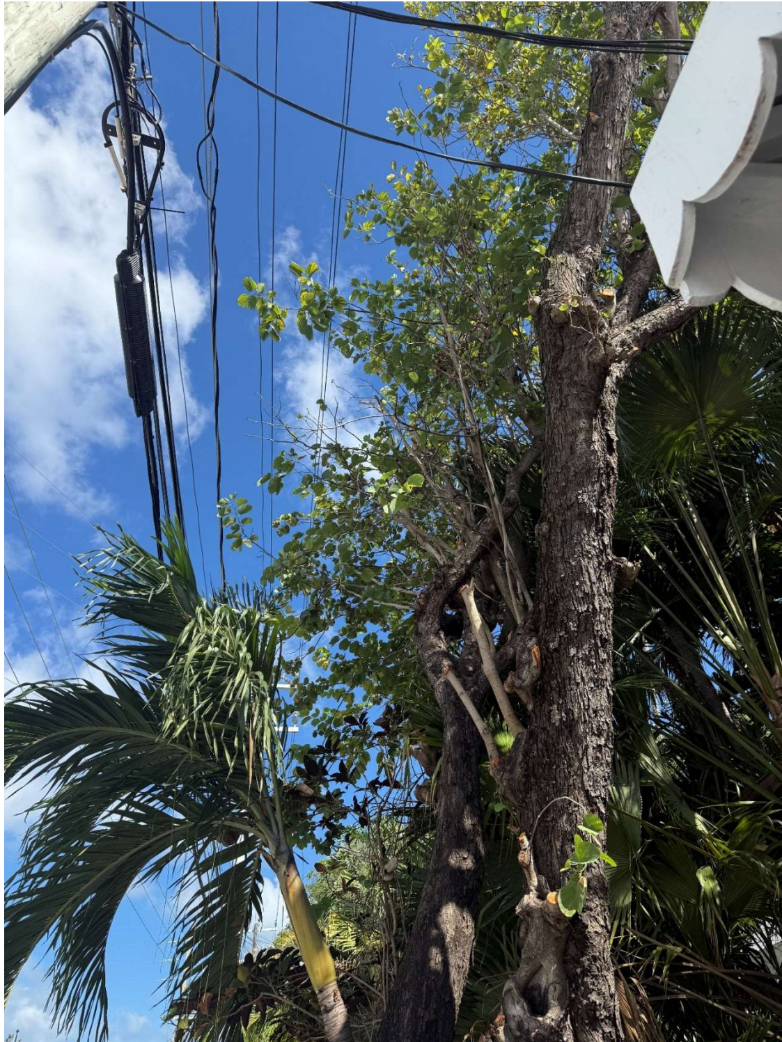
Tree has clear evidence of past and present termite infestation.
